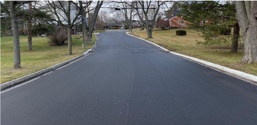
Latham after Mill and Overlay – Rating 9
