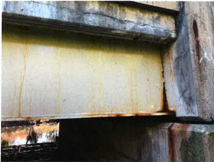
Document Name: IMG_2108.JPG Category: Superstructure Span Number: Comments: Rust Staining at Stringer Ends
