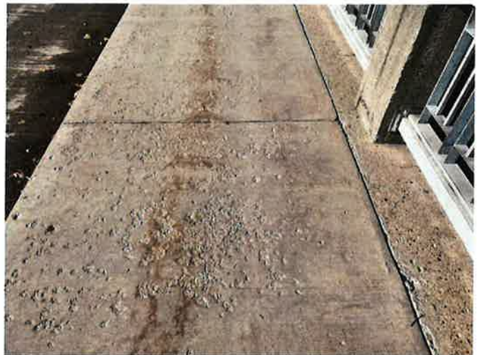
Document Name: IMG_2096.JPG Category: Deck Span Number: Comments: North Sidewalk Surface Pitting
