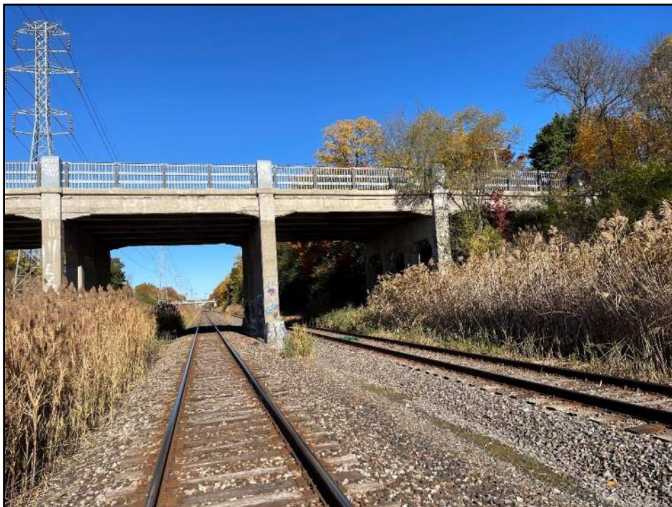
Southeast bridge elevation
