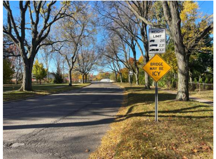
Document Name: IMG_7226.JPG Category: Posting Span Number: Comments: Westbound posting sign
