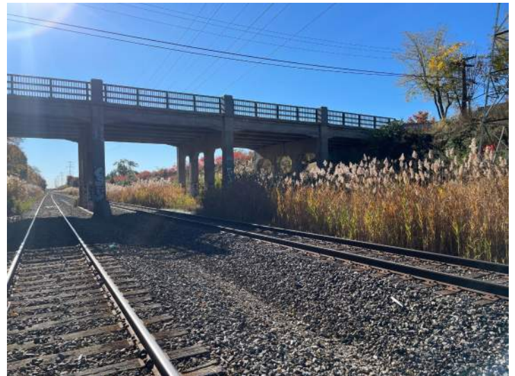
Document Name: IMG_7269.JPG Category: Elevation Span Number: Comments: NW bridge elevation
