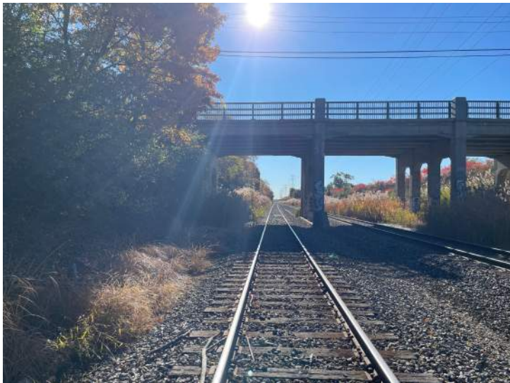
Document Name: IMG_7268.JPG Category: Elevation Span Number: Comments: NE bridge elevation
