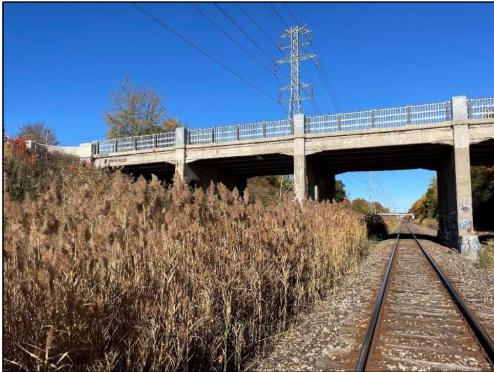
Southwest bridge elevation
