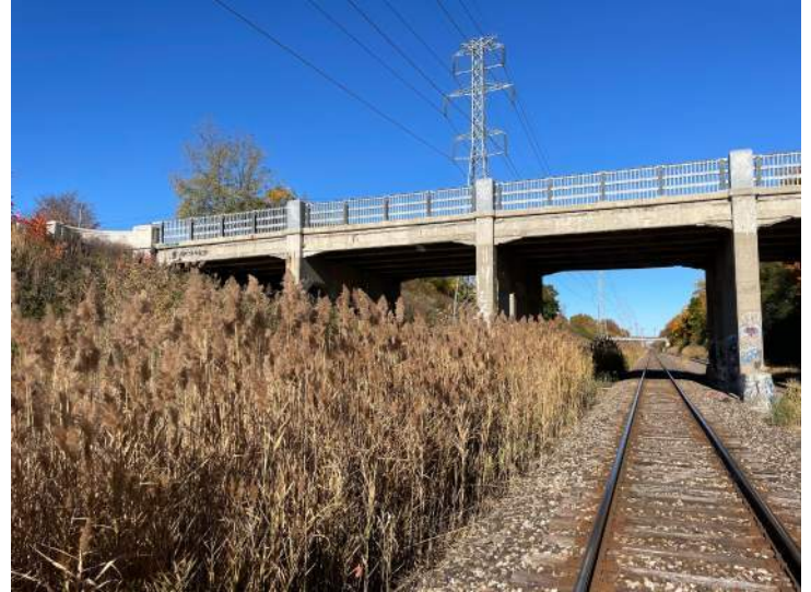
Document Name: IMG_7267.JPG Category: Elevation Span Number: Comments: SW bridge elevation
