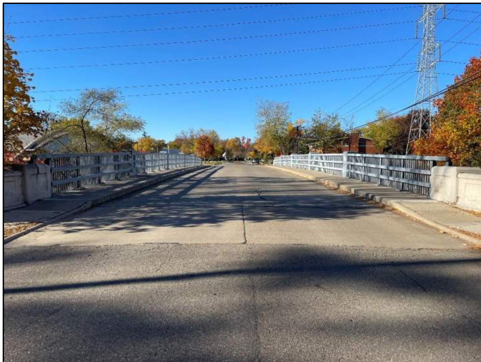
Bridge alignment, looking southwest
