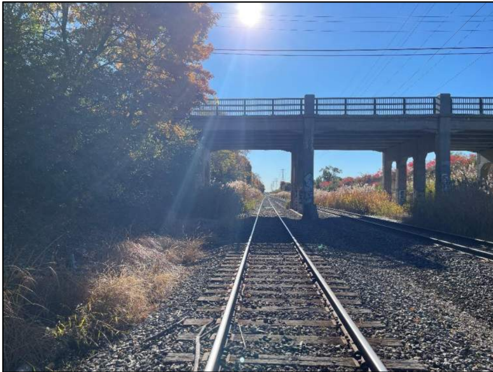
Northeast bridge elevation
