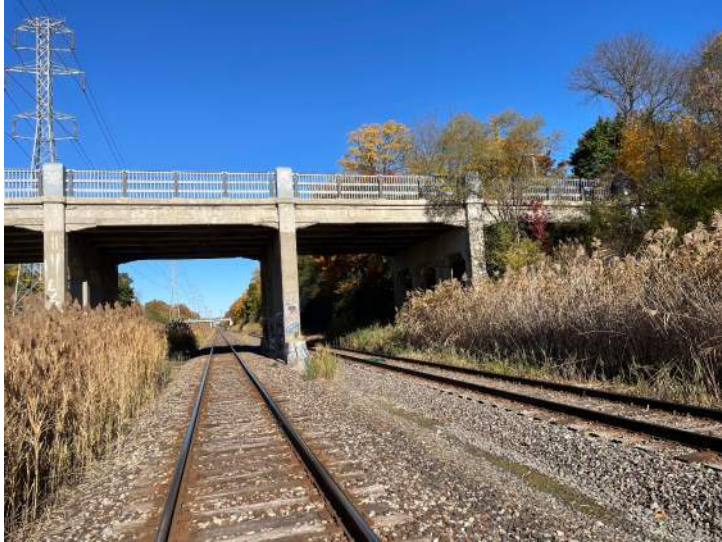
Document Name: IMG_7266.JPG Category: Elevation Span Number: Comments: SE bridge elevation
