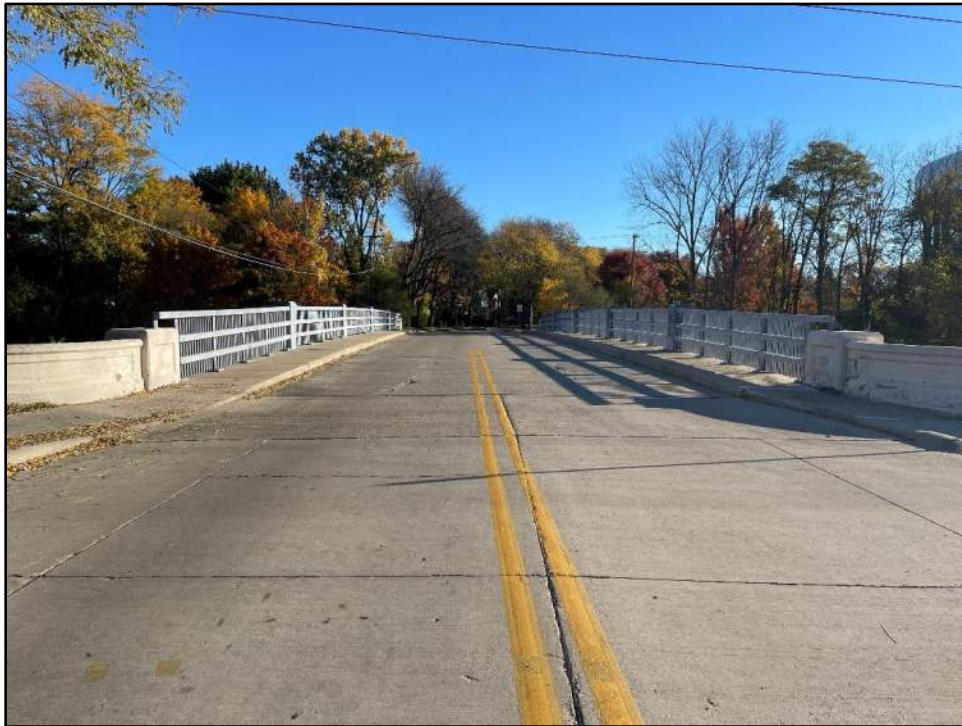
Bridge alignment, looking northeast
