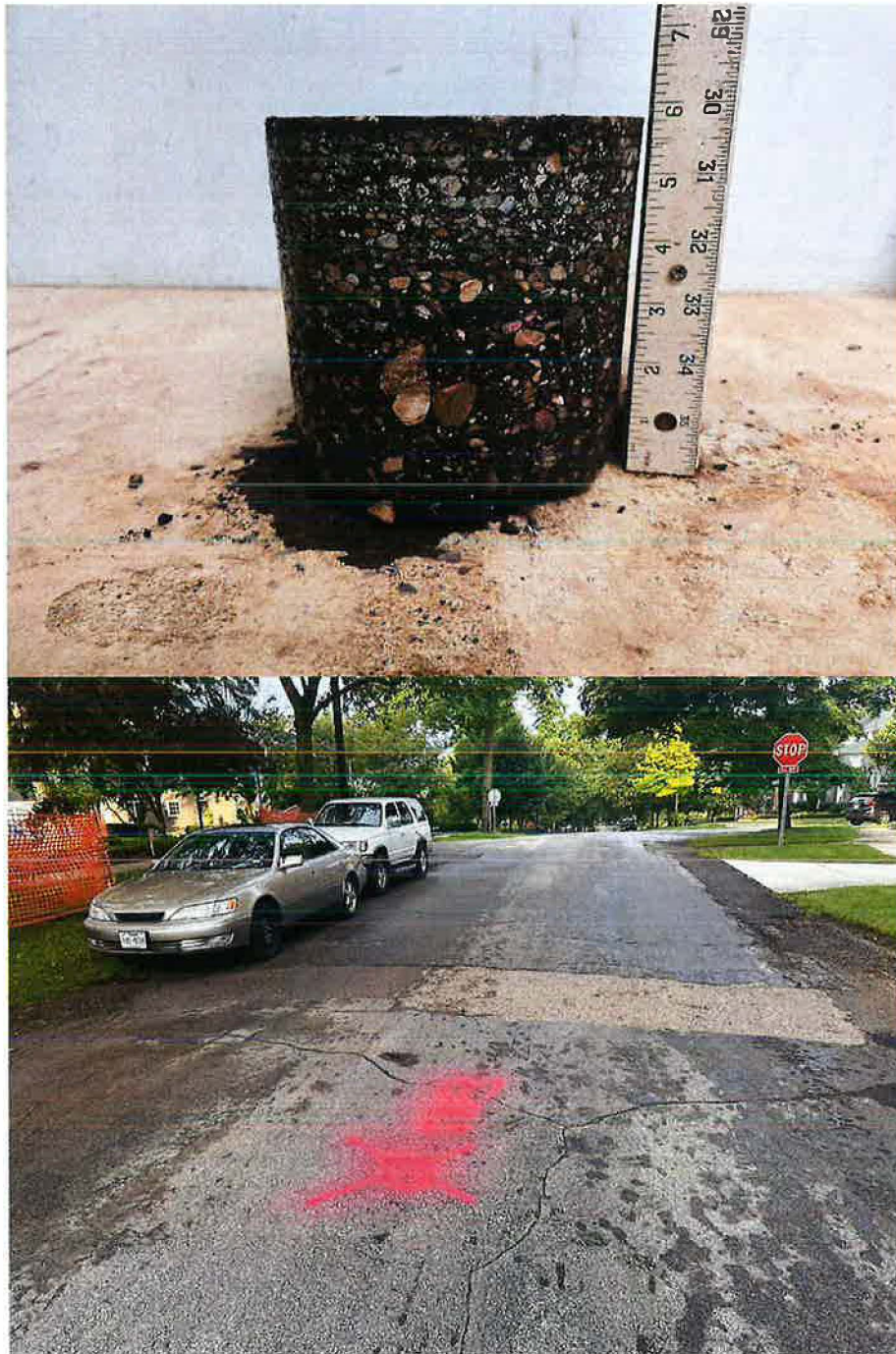
Core Photograph of SB-3: Bituminous Concrete = 5-3/4 inches
