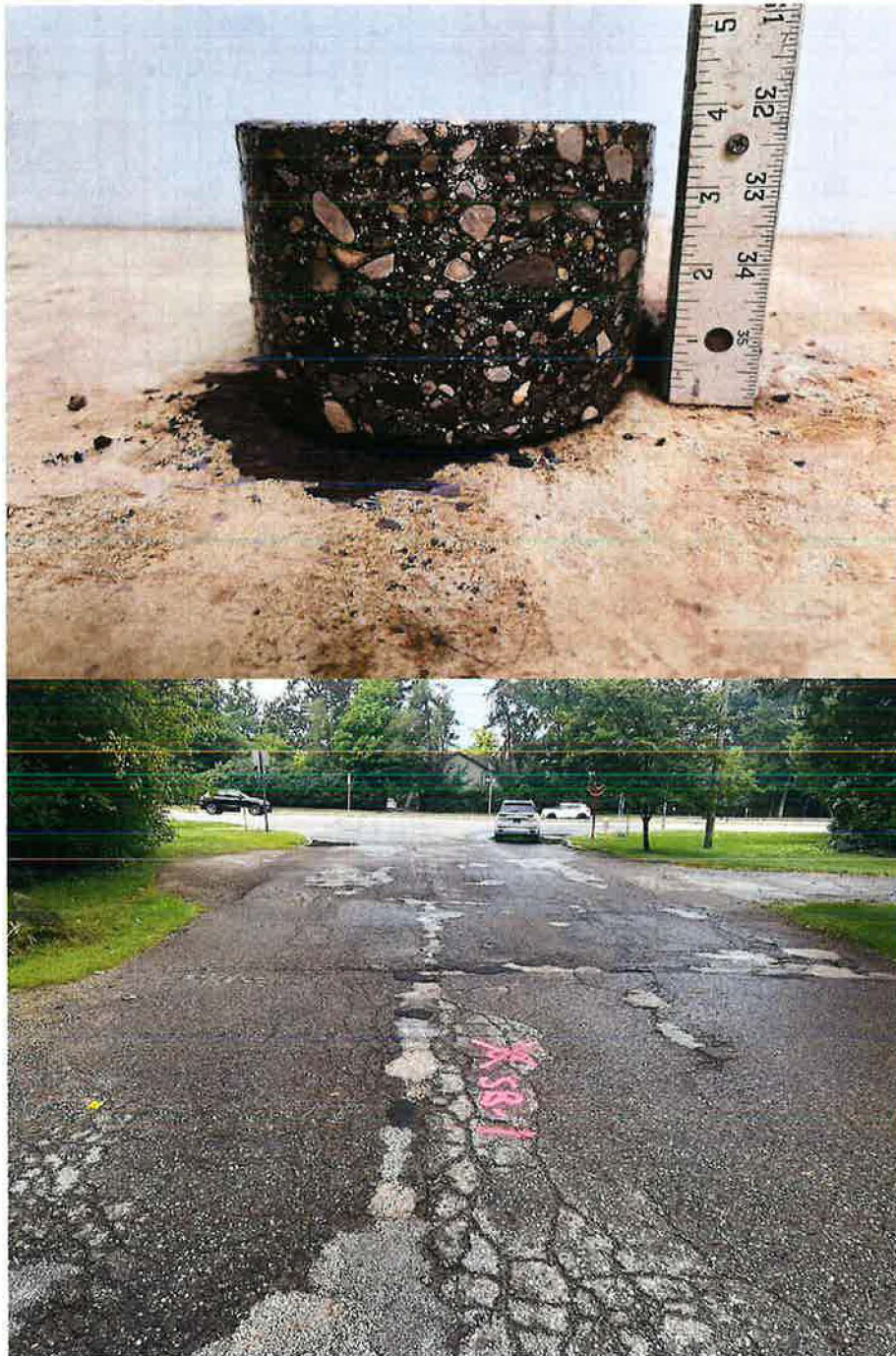
Core Photograph of SB-1: Bituminous Concrete = 3-3/4 inches
