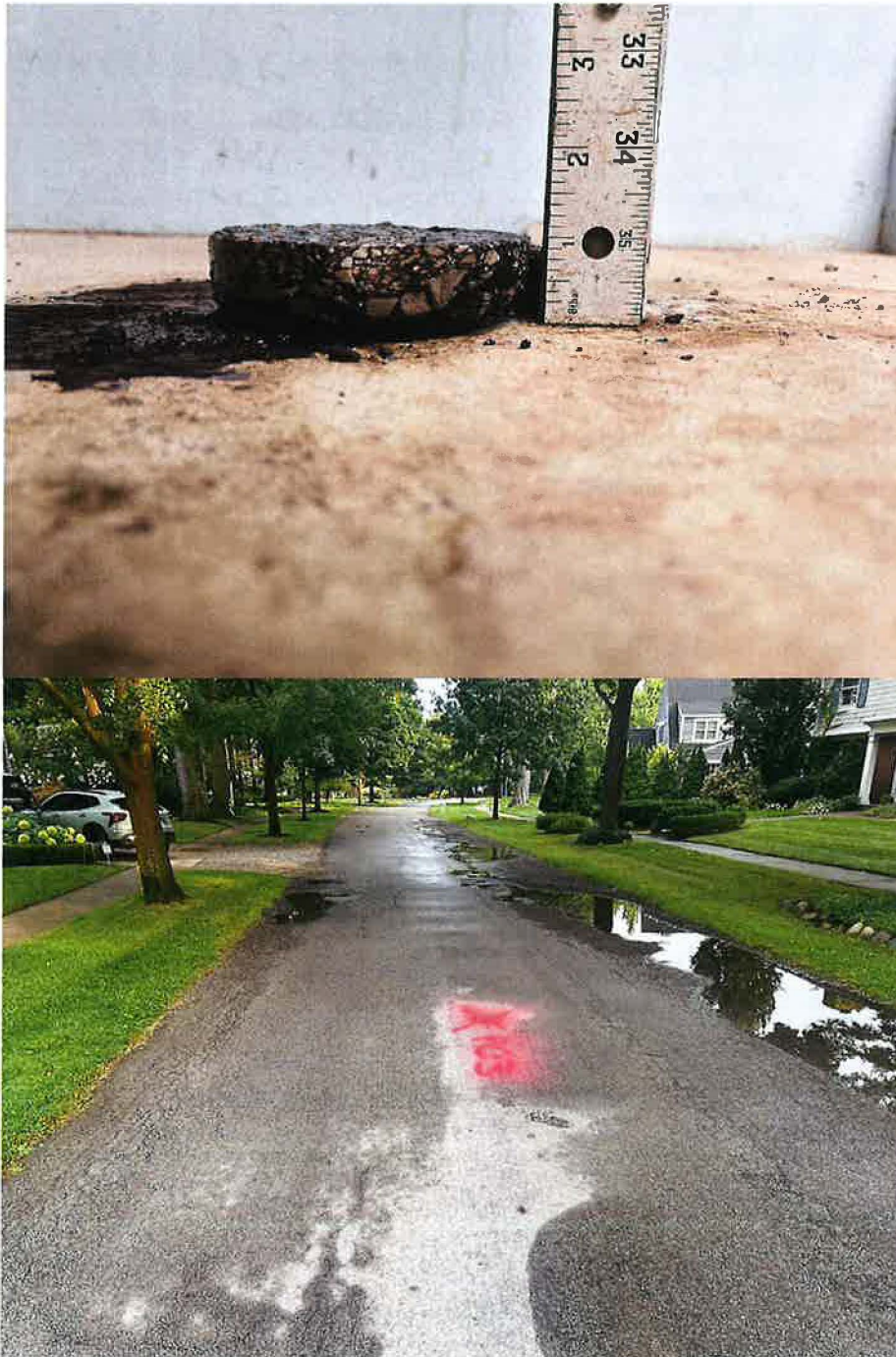
Core Photograph of PC-3: Bituminous Concrete = 1 inch
