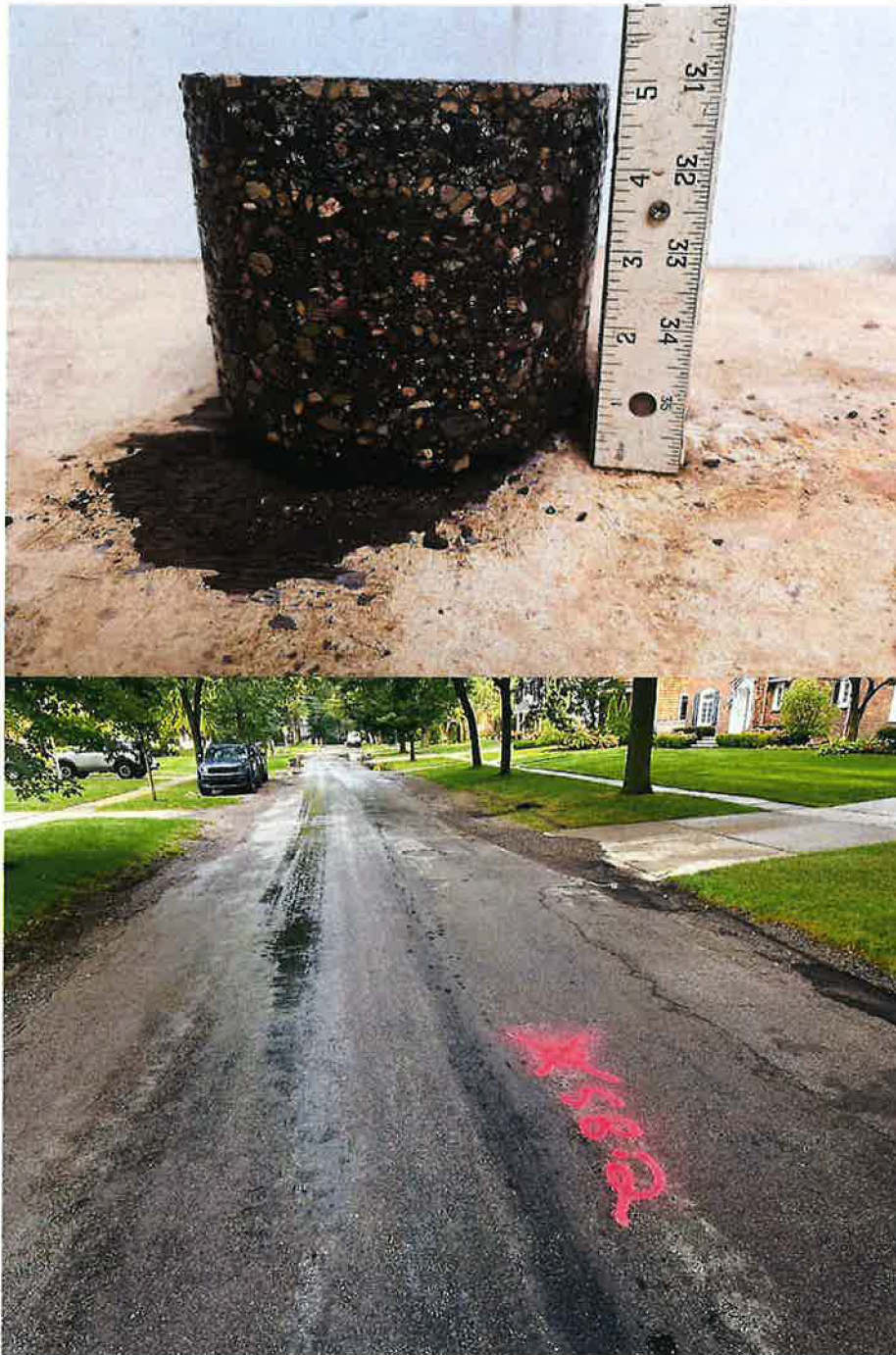
Core Photograph of SB-2: Bituminous Concrete = 5 inches
