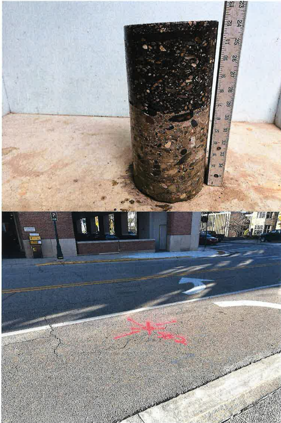
Core Photograph of B-2: HMA Pavement = 5 inches PCC Pavement = 7 inches
