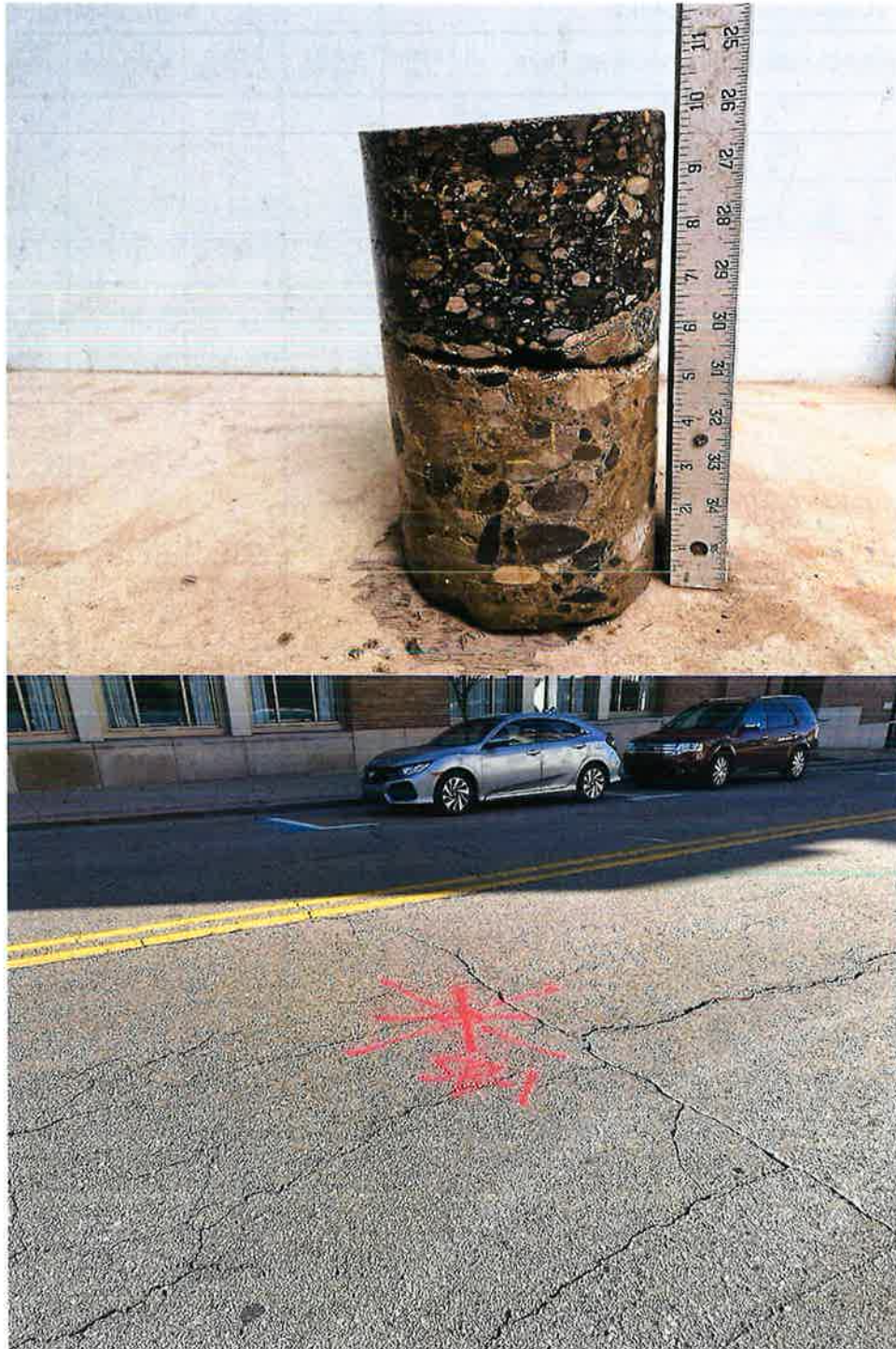
Core Photograph of B-1: HMA Pavement = 4-1/2 inches PCC Pavement = 5-1/2 inches
