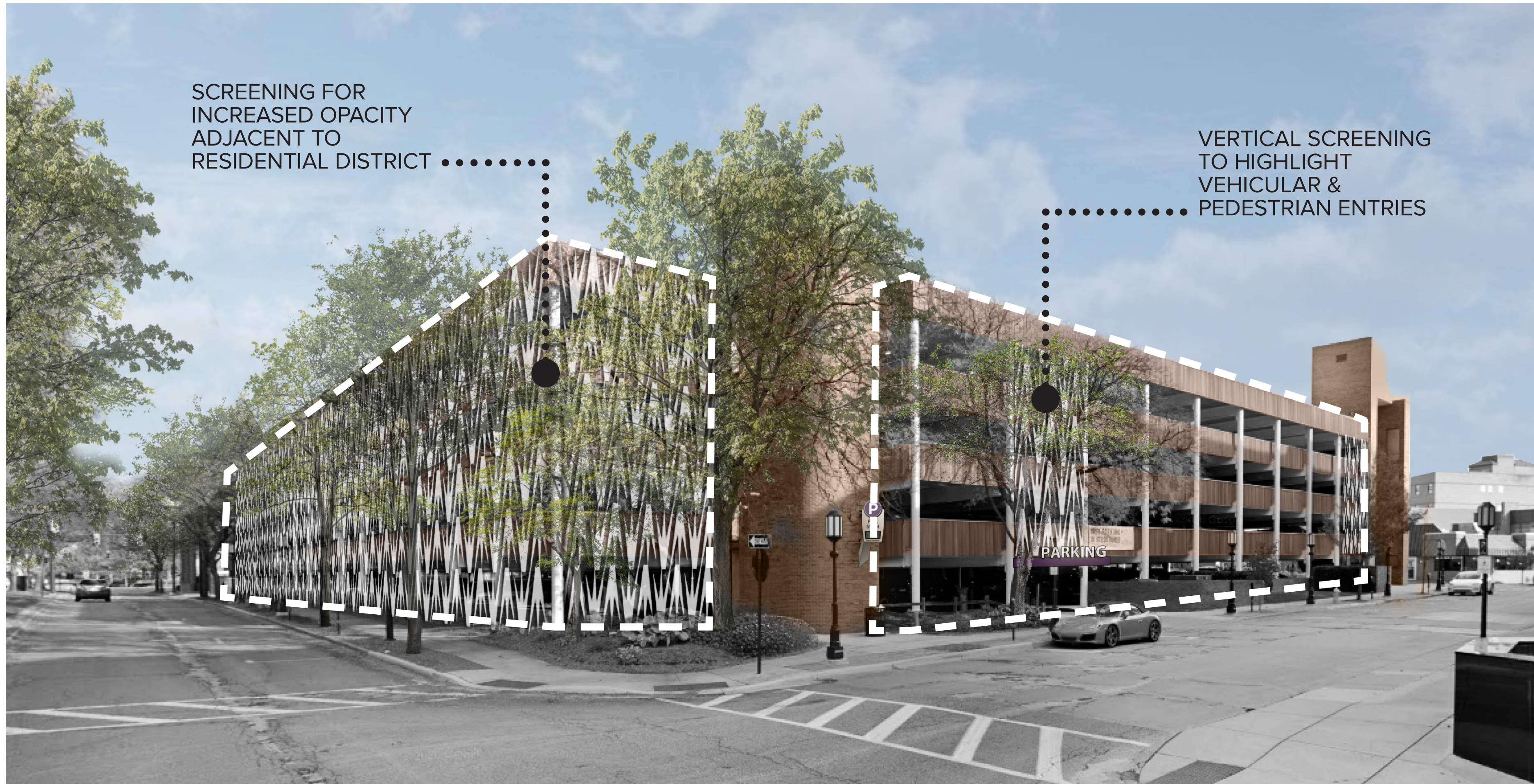
FACADE 2 - REPLACED ALUMINUM PANELS W/ PATTERNED SCREENING
