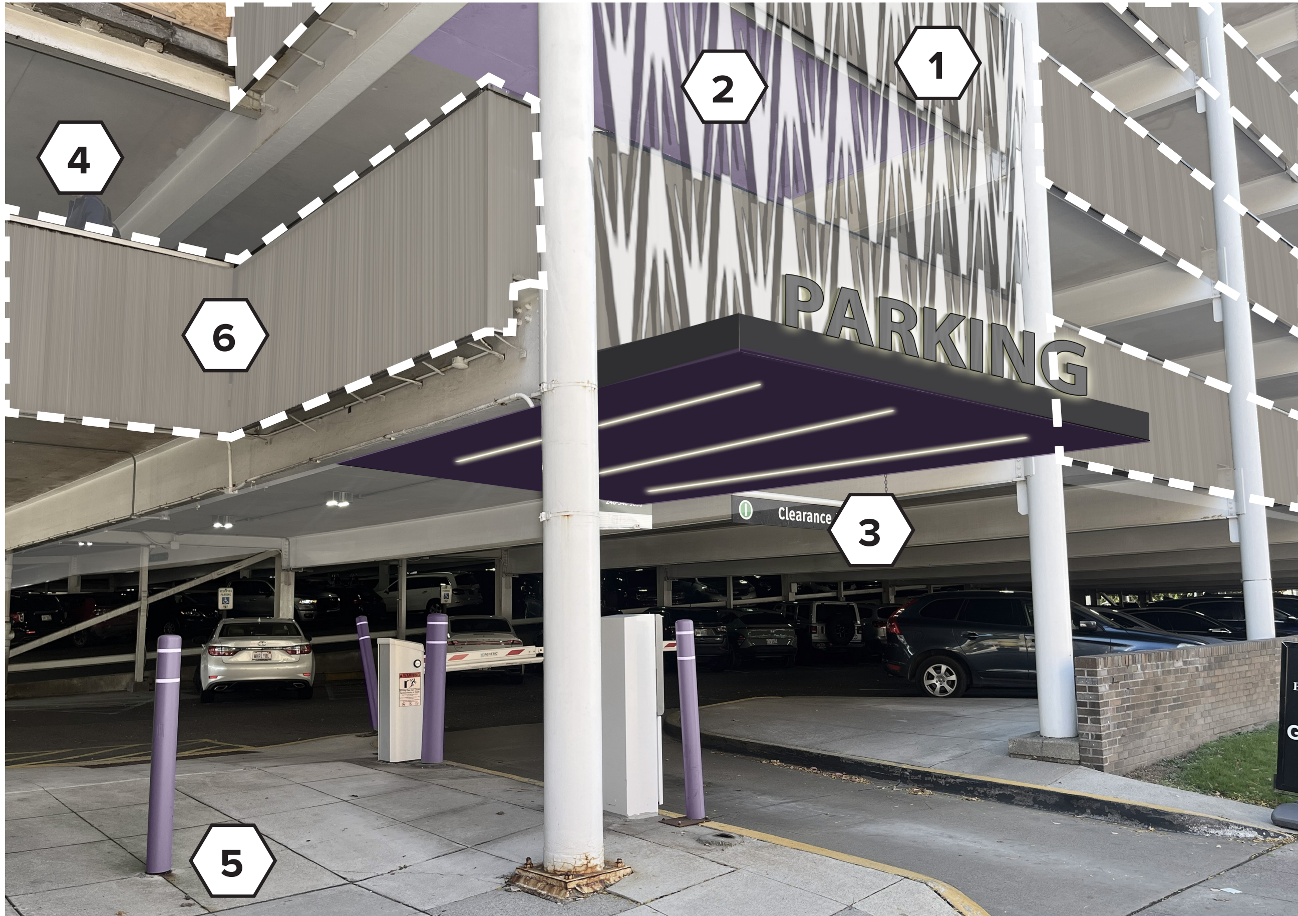
VEHICULAR ENTRY AT PARK STREET
