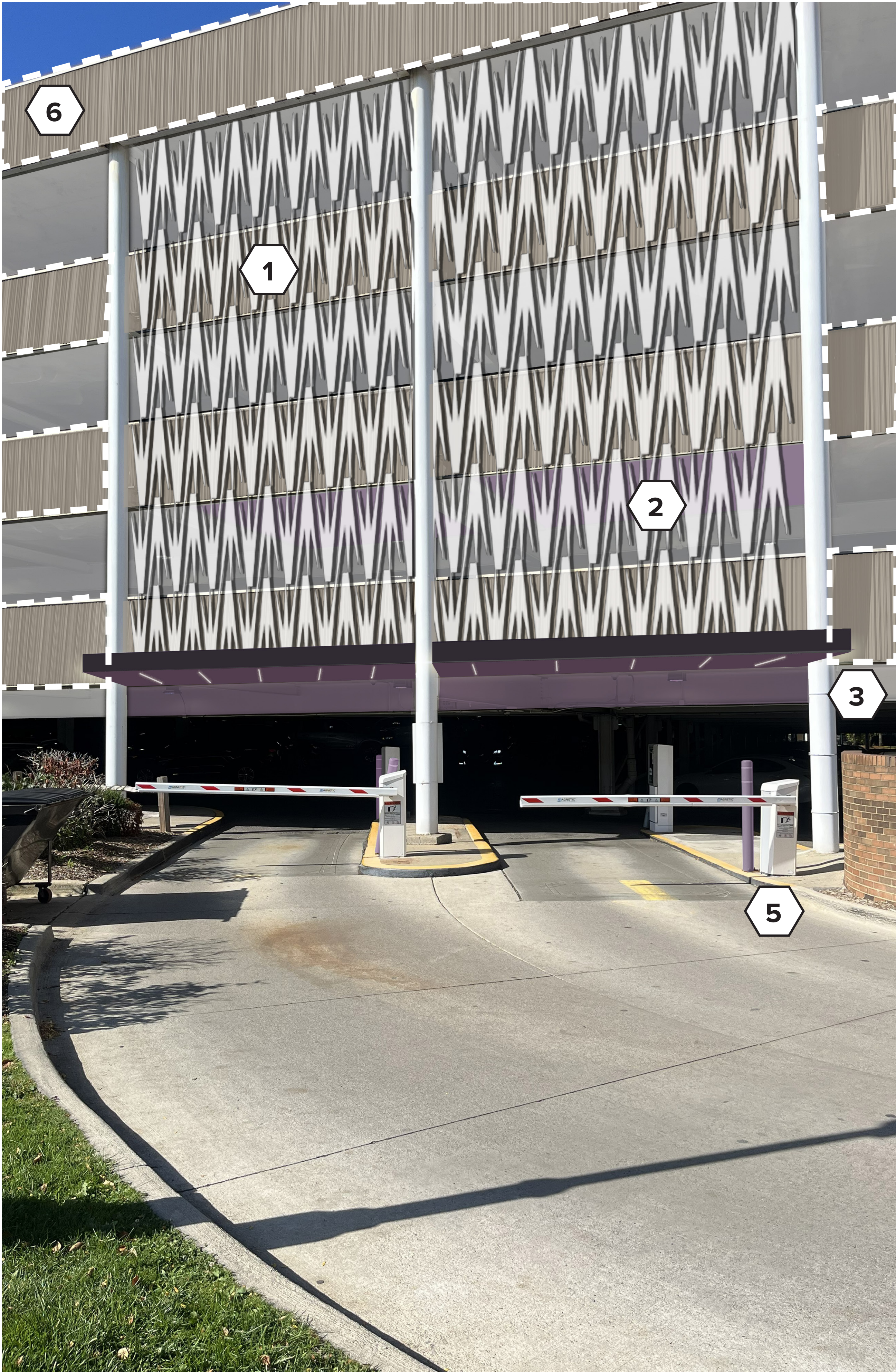
VEHICULAR EXIT AT PARKING LOT
