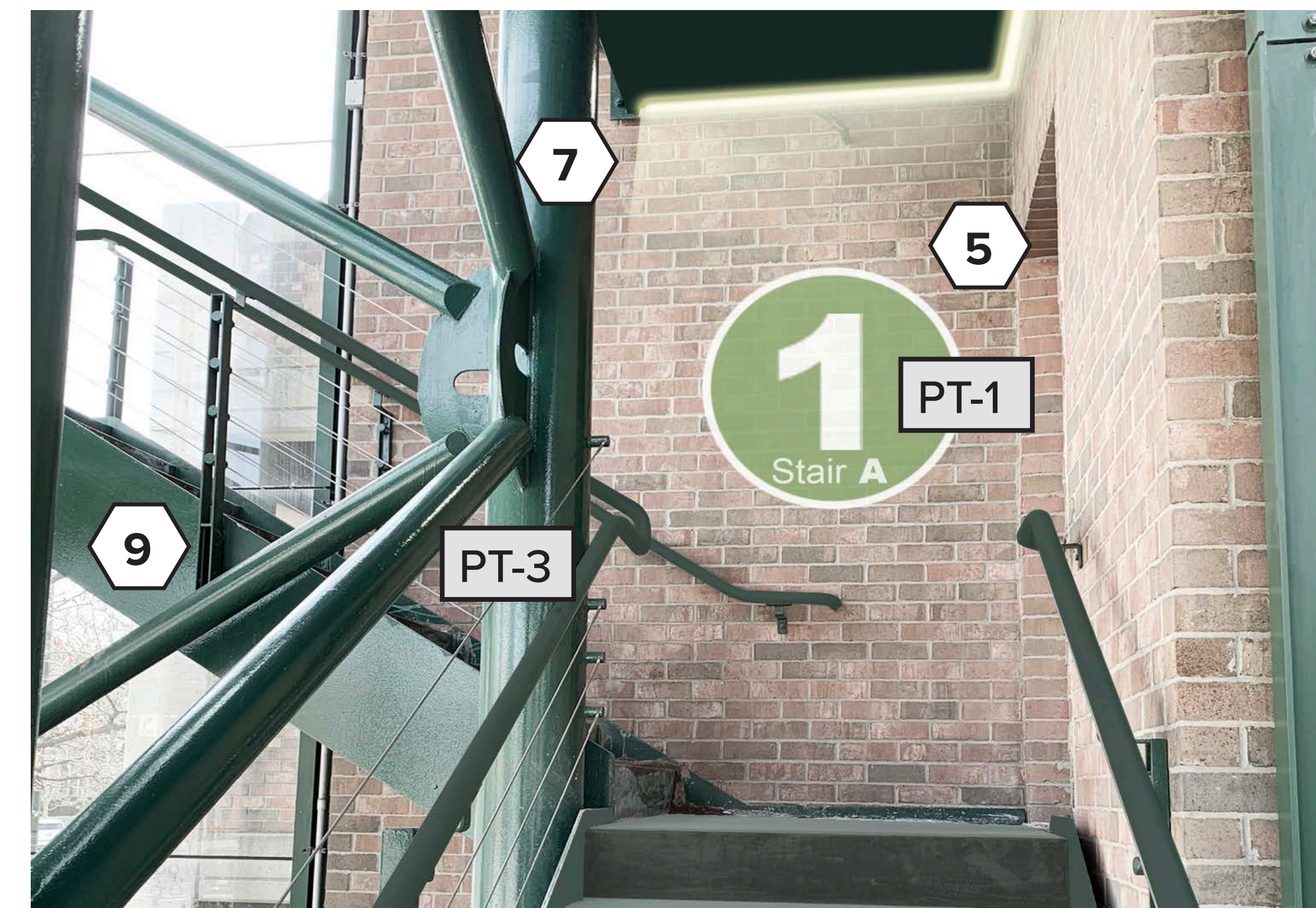
STAIR A INTERIOR
