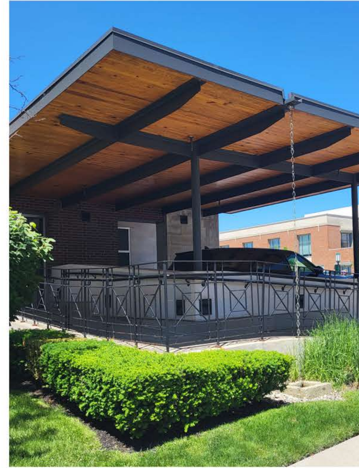
Steel roof with wooden ceiling
