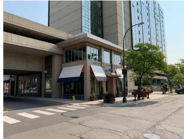
Existing Awnings – NE Corner
