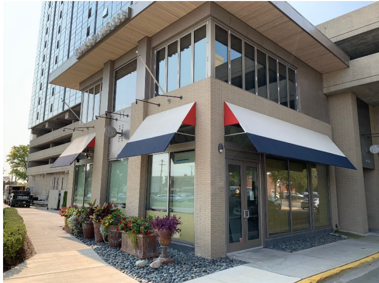
Existing Awnings – SW Corner
