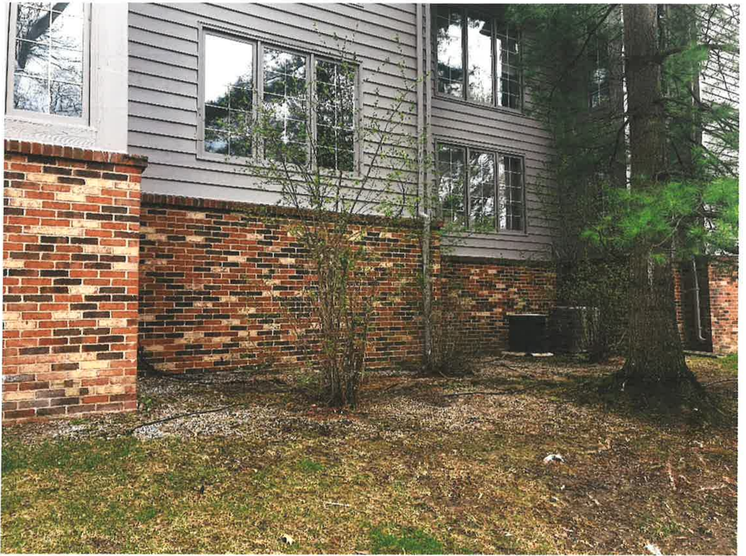
752 Hidden Ravines Trail Neighbors AC units
