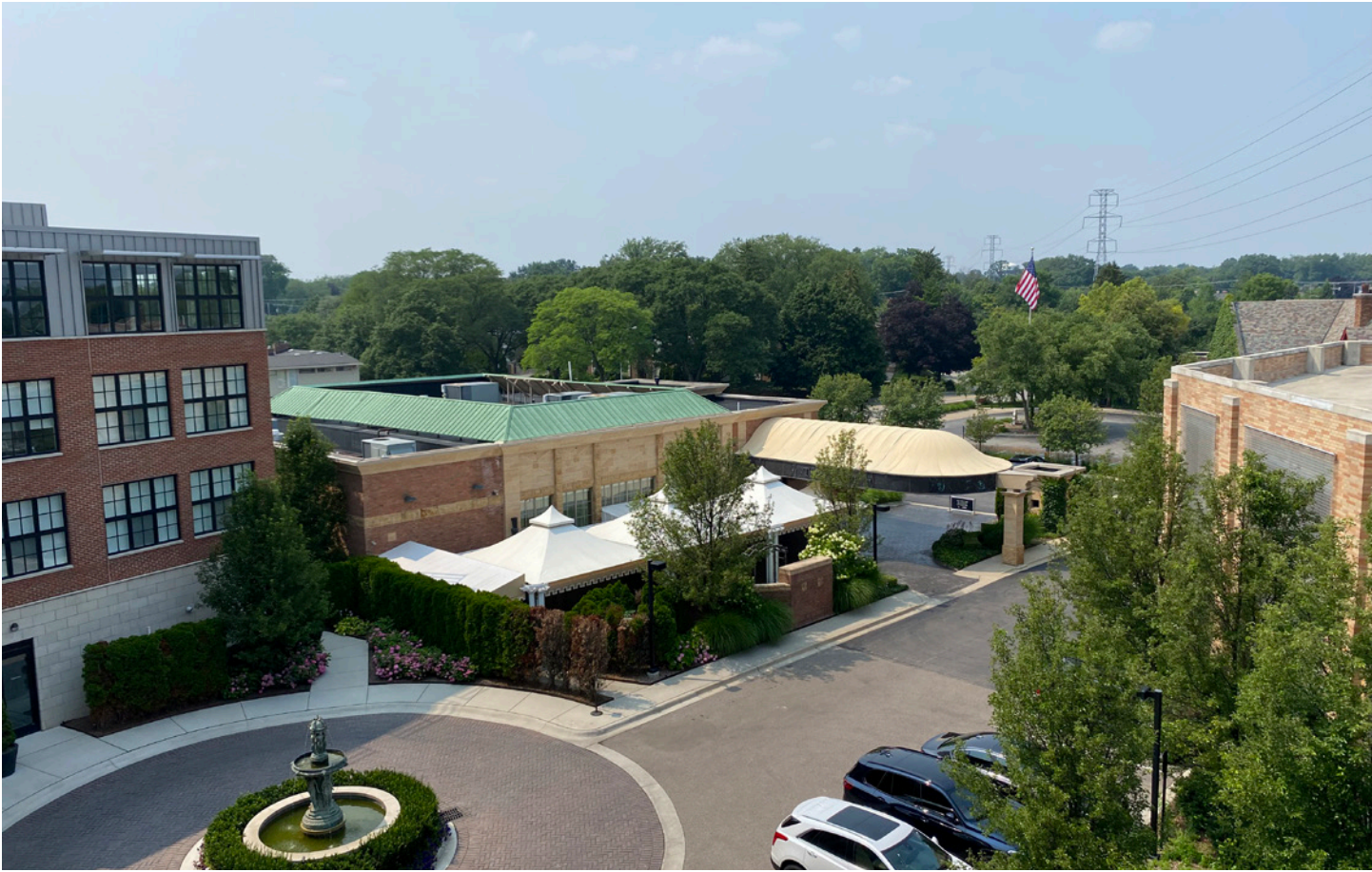
Aerial Photograph - East Facade
