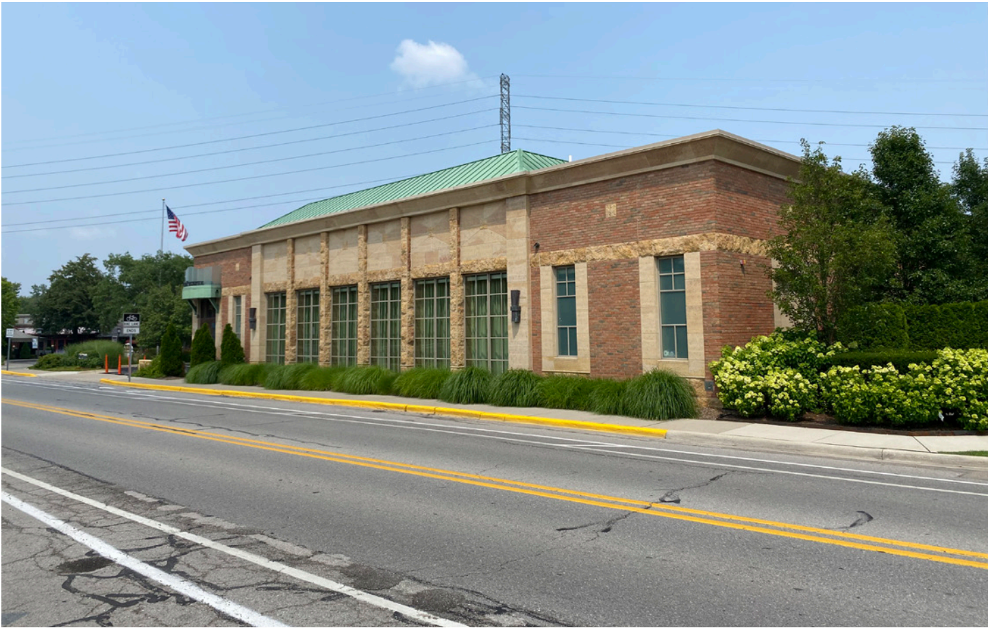
South Eton Street
