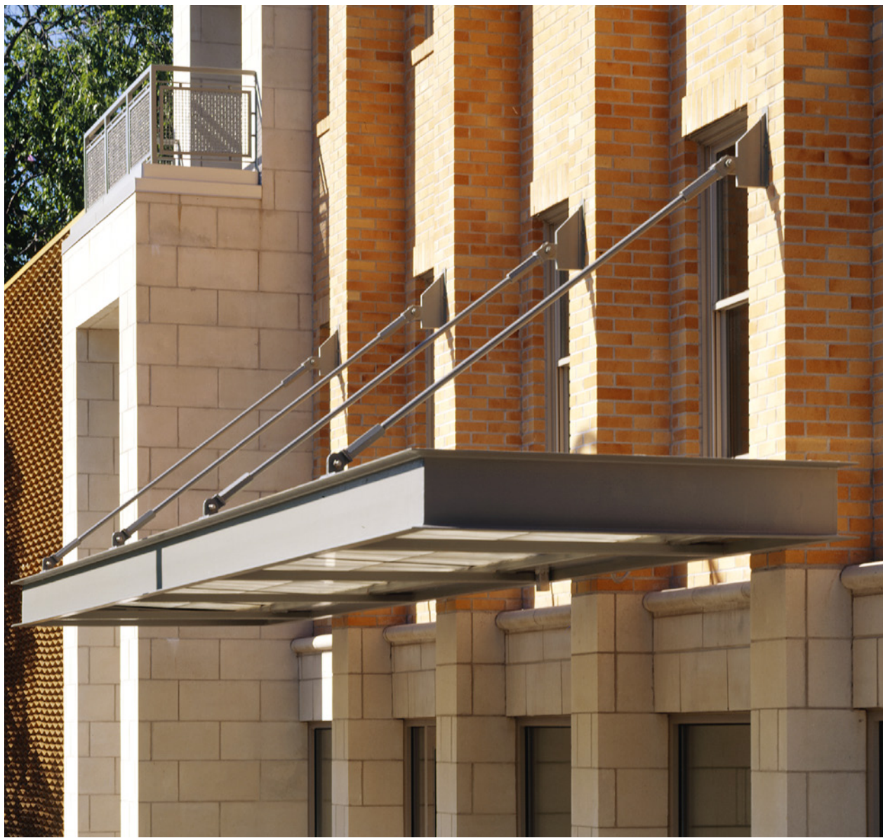
Steel and Glass Canopy
