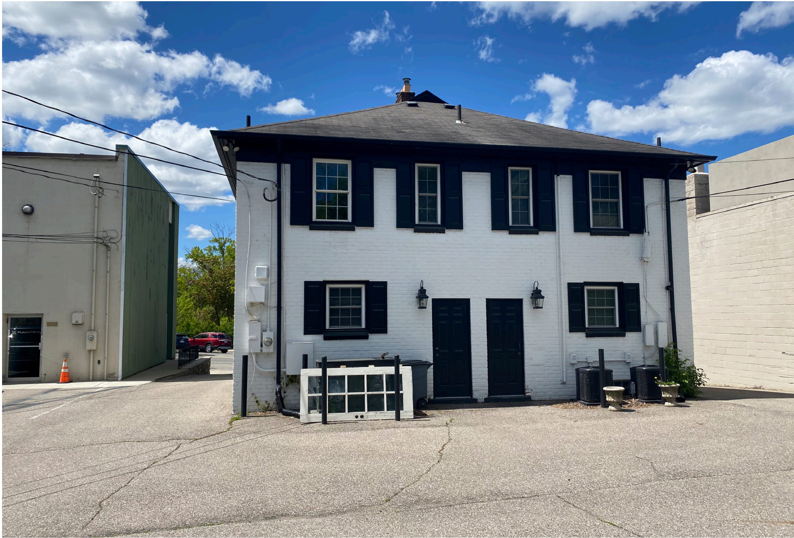
H5 A012 Photographs - Existing Site SCALE: 1" = 10'-0"
