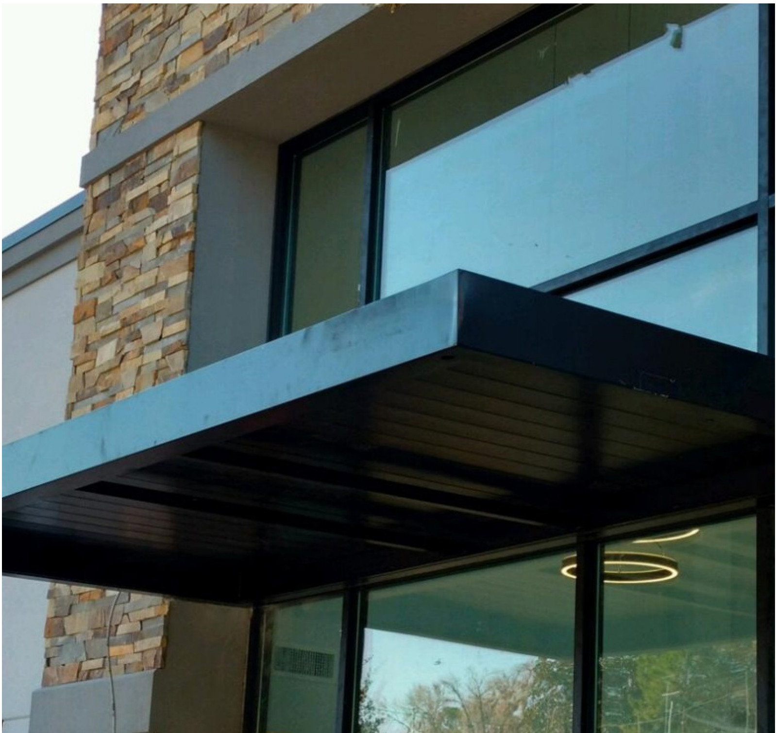
Steel Entrance Canopy (Cantilevered) Black Finish
