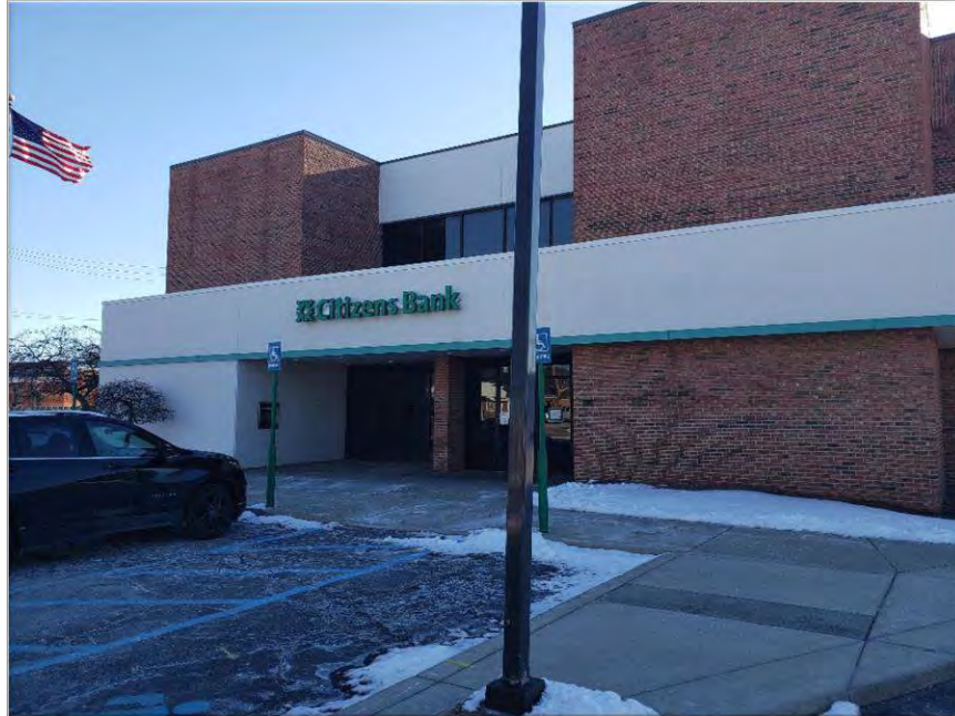
View of subject site, looking south
