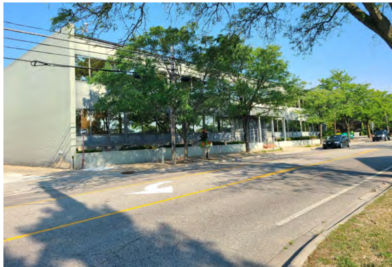
Adams @ Alley (SE Corner) looking North
