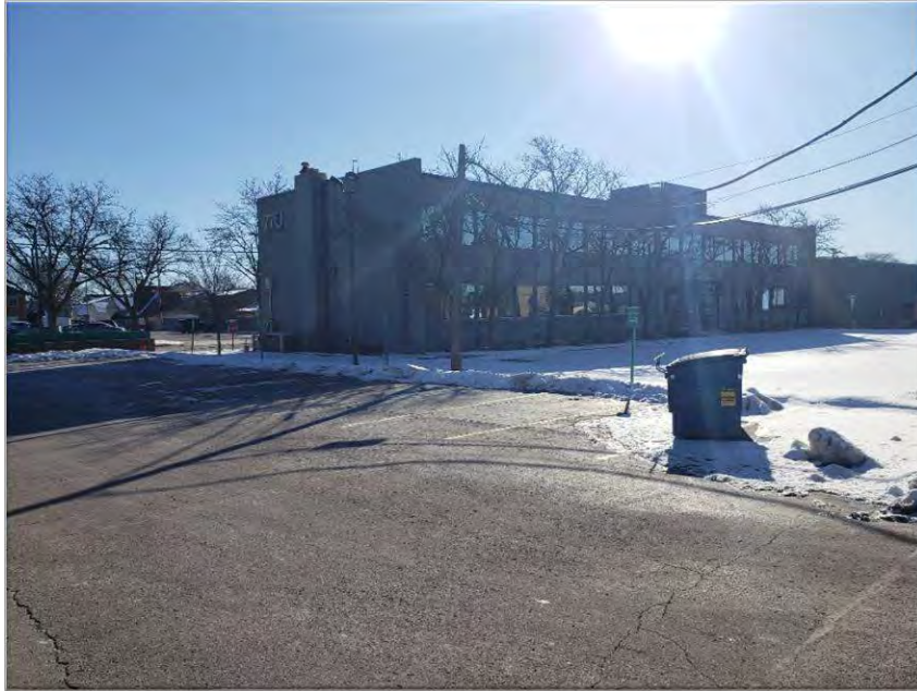
View southwest of the subject site (adjoining office building)
