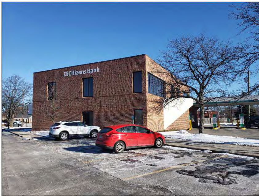
View of the subject building from the southwest
