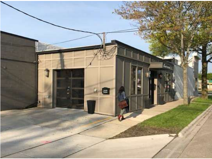
Figure 53. Building with potential for sleeve activation.
