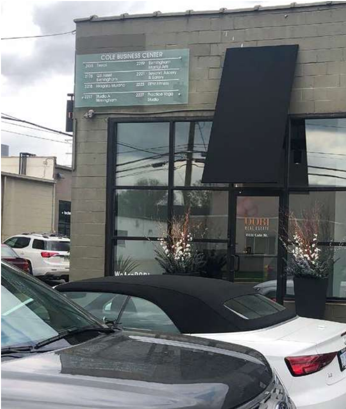
Figure 58. Current conditions in the Lower Rail District.
