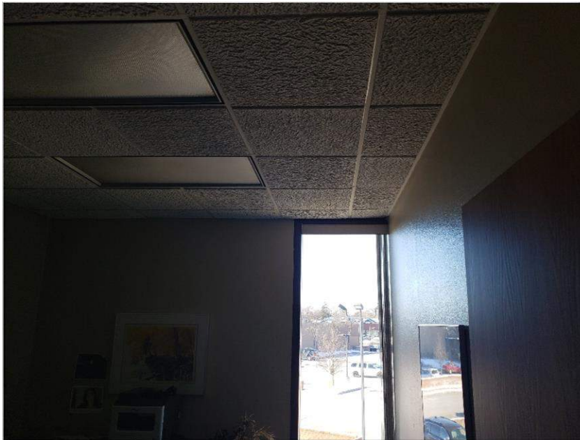
Office finishes (typical)
