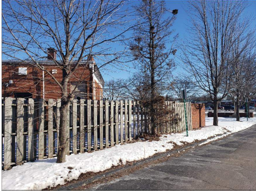
View north of subject site property (Plant Store/former Gas Station)
