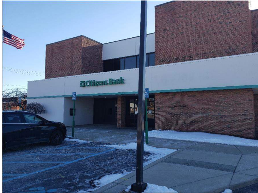
View of subject site, looking south
