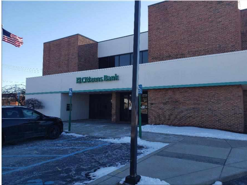
View of subject site, looking south
