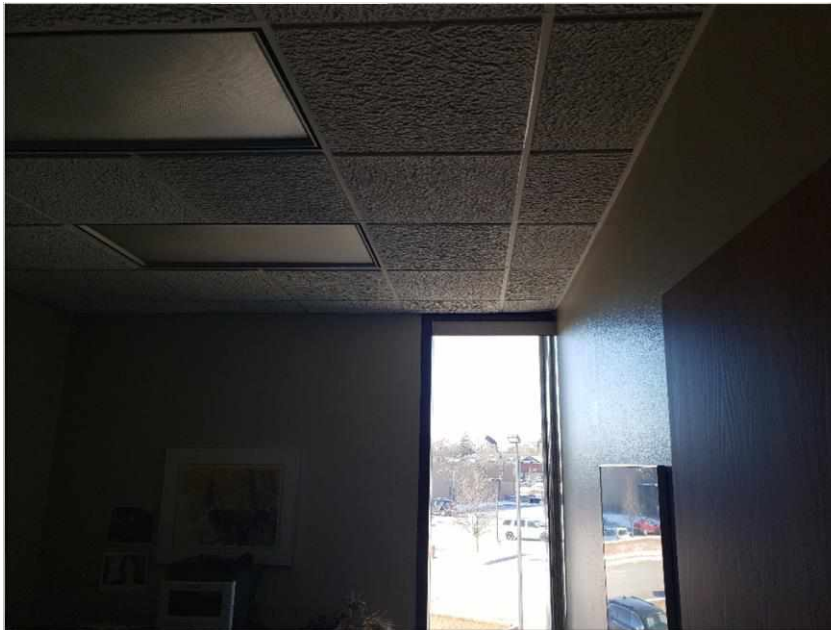
Office finishes (typical)
