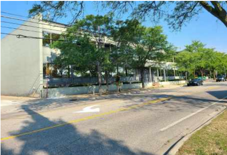
Adams @ Alley (SE Corner) looking North
