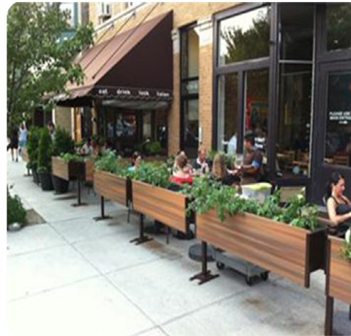
Figure 2. Wood and metal planters as a barrier.
