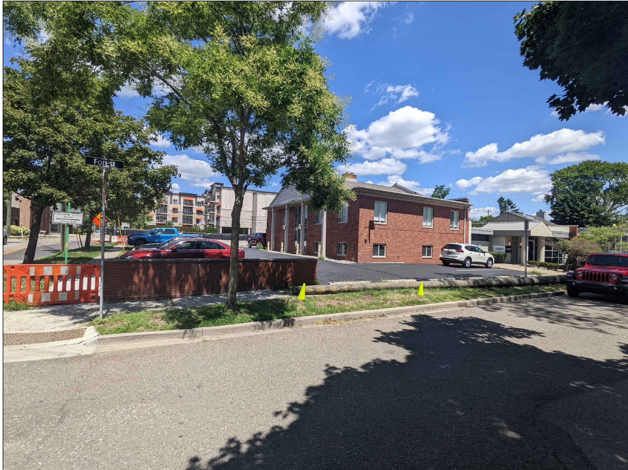
EXISTING SOUTH SIDE OF SITE LOOKING NORTH
