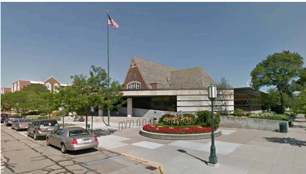
Figure 46. The Library's entrance plaza.
