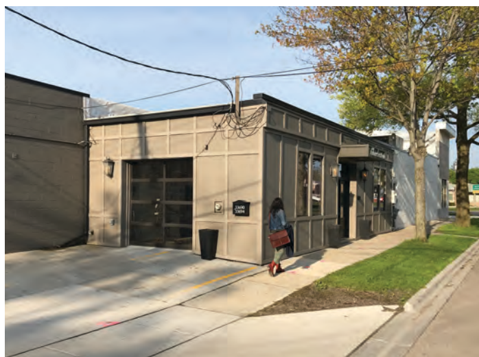
Figure 54. Building with potential for sleeve activation.
