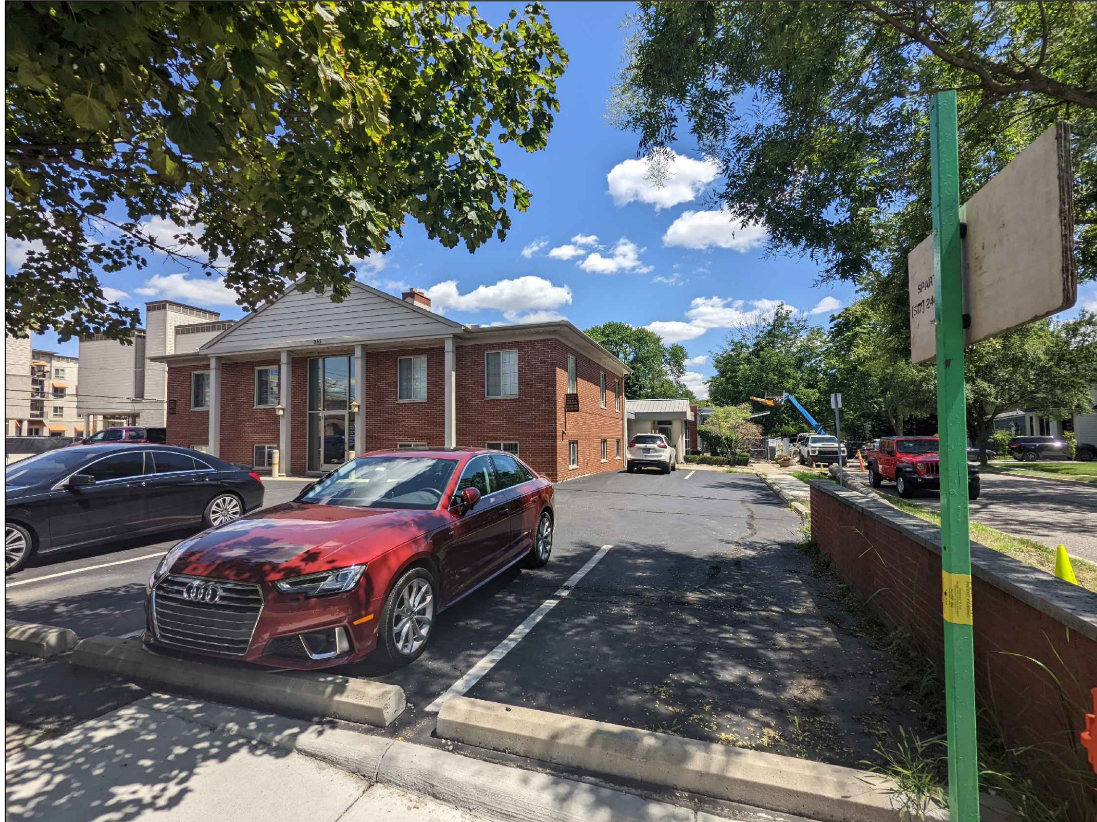
EXISTING SOUTH-WEST PART OF SITE (LOOKING EAST)
