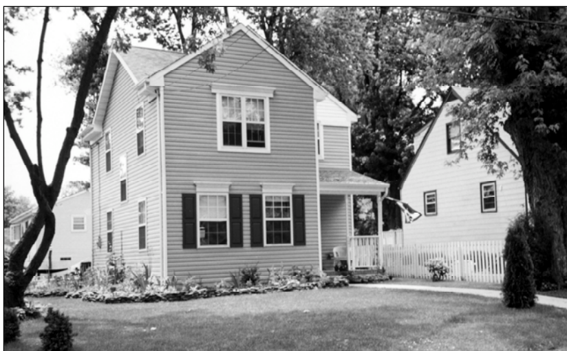
In Wall Township in Monmouth County, New Jersey, the affordable housing initiative has used infill housing to create more affordable housing opportunities.
