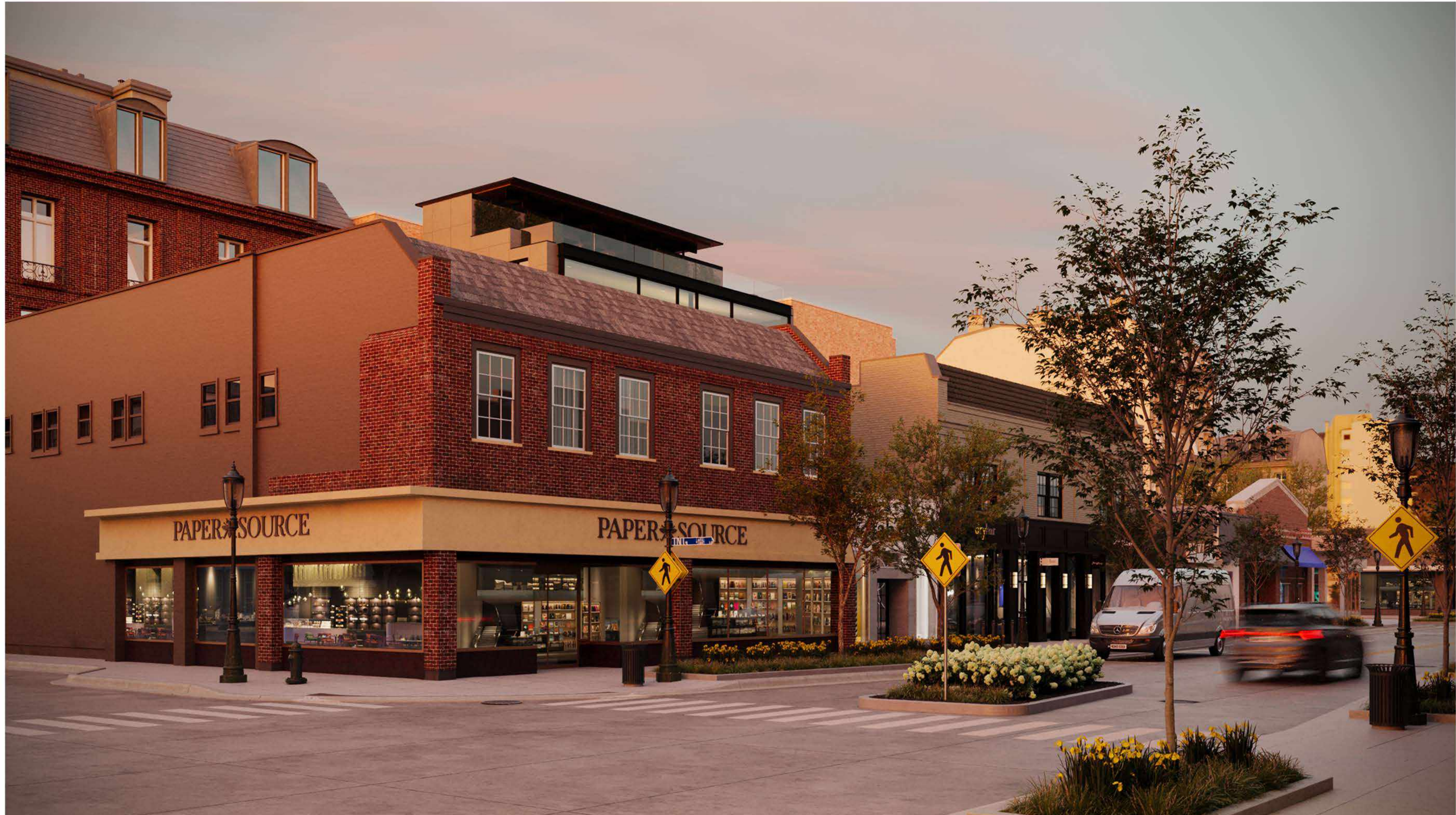
PIERCE STREET WITH MAPLE ROAD VIEW SUNSET
