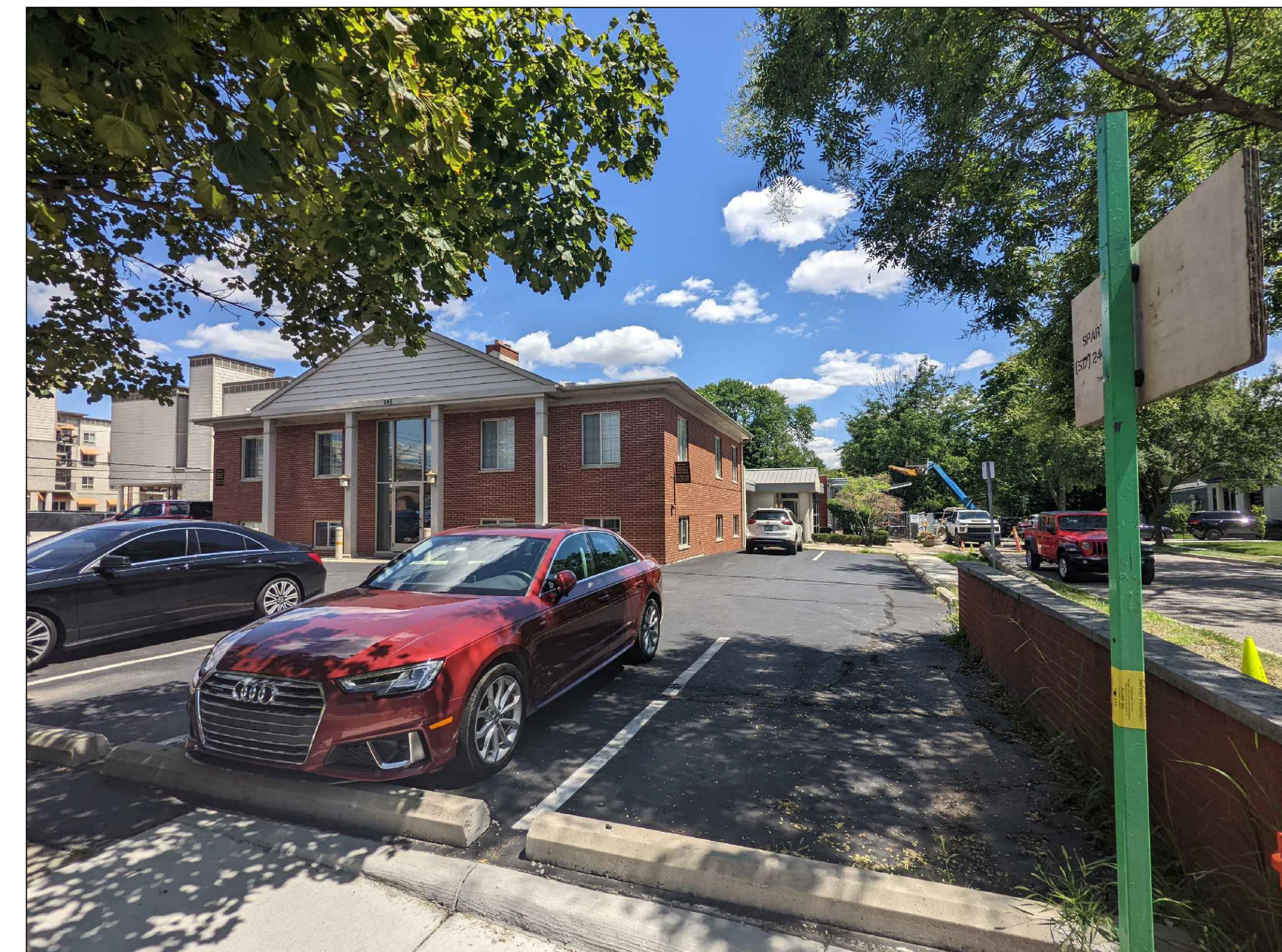
EXISTING SOUTH-WEST PART OF SITE (LOOKING EAST)
