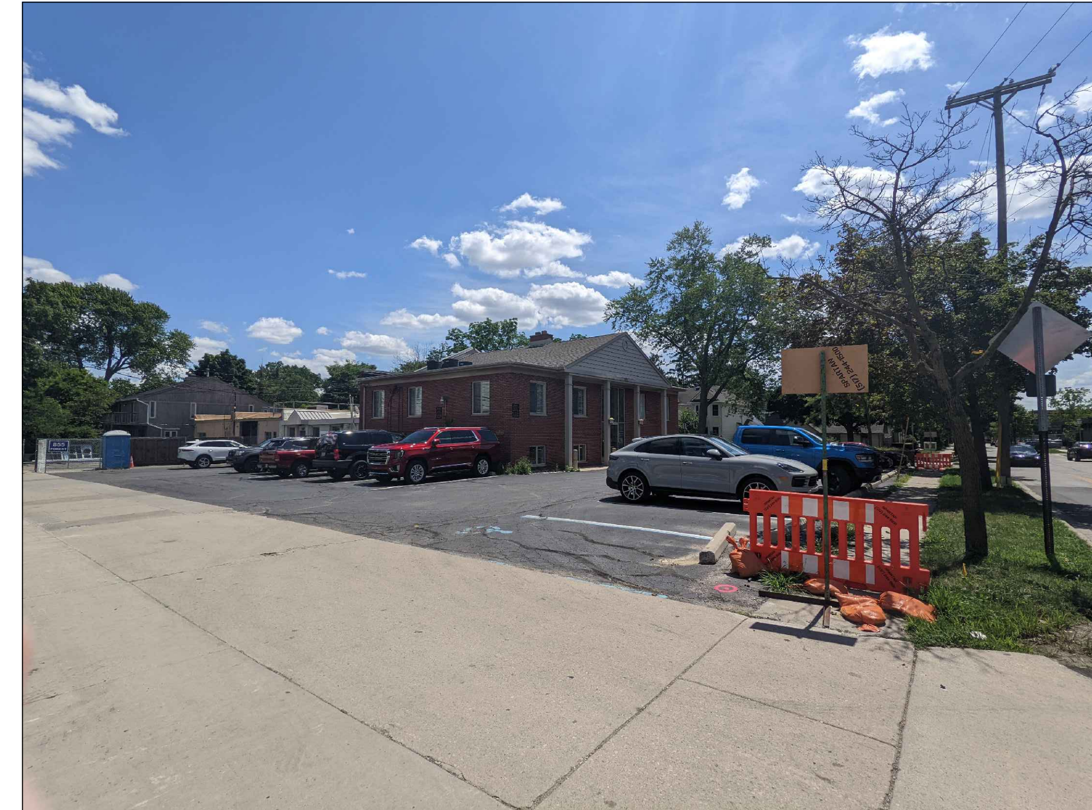
EXISTING ALLEY / NORTH WEST PART OF SITE (LOOKING SOUTH-EAST)
