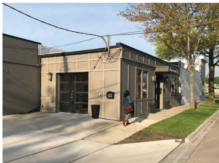
Figure 54. Building with potential for sleeve activation.
