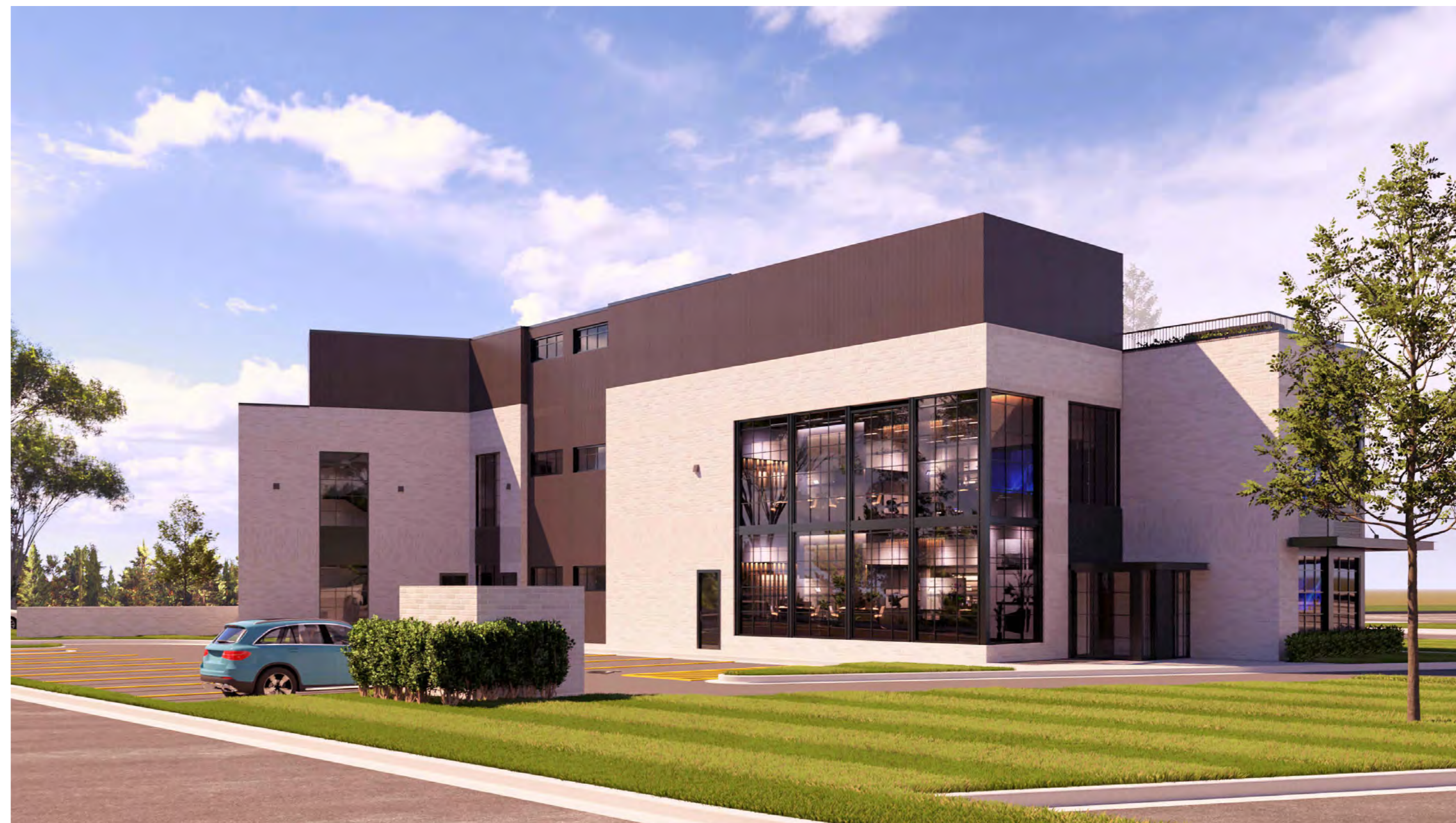
View of West facade from public alley
