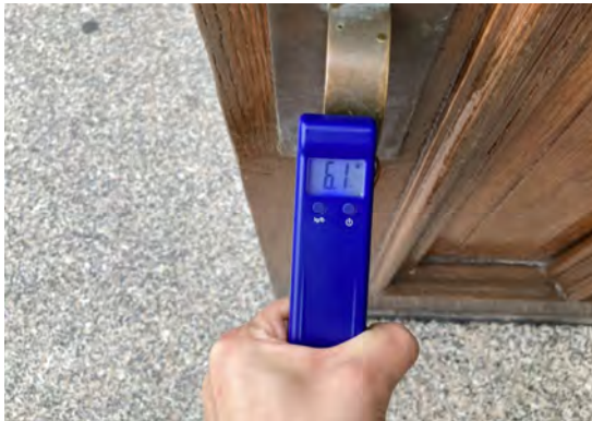
IMAGE 4.2.03 NORTH FRONT ENTRY DOOR
