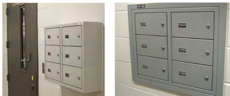
Figure 7.2: Surface mounted and recessed Gun Lockers
