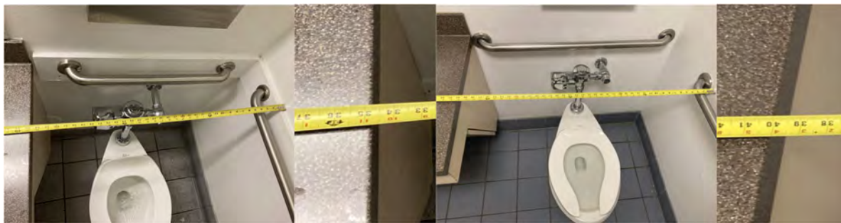
4.2.33 - LOWER LEVEL AND 2ND FLOOR UNISEX WATER CLOSET CLEARANCE
