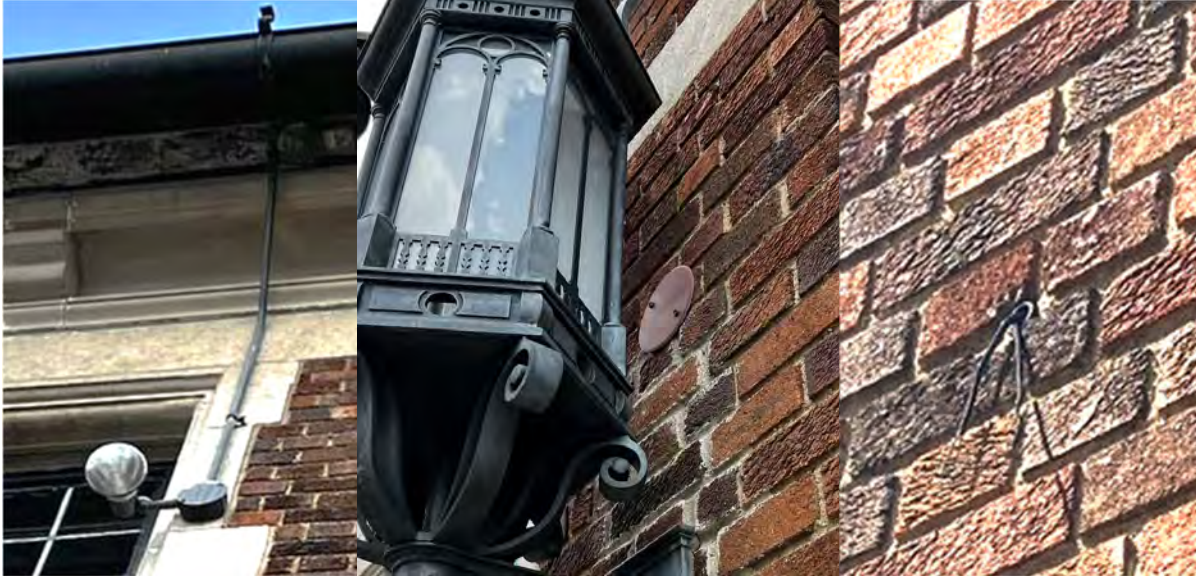
IMAGES 3.1.18 EXPOSED CONDUIT ABANDONED SECURITY LIGHT, ELECTRICAL COVER PLATE, AND FACADE HOLE
