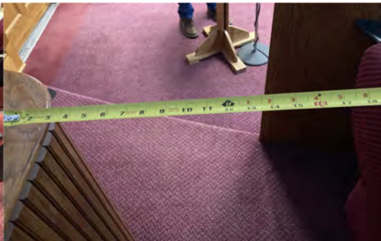
IMAGES 4.2.16 - COMMISSION ROOM WHEELCHAIR SPACE AT CLERK AND PLATFORM CIRCULATION
