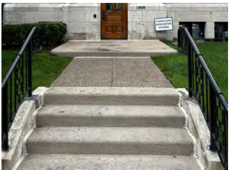
IMAGE 4.1.07 SIDE WEST EXTERIOR STAIRS
