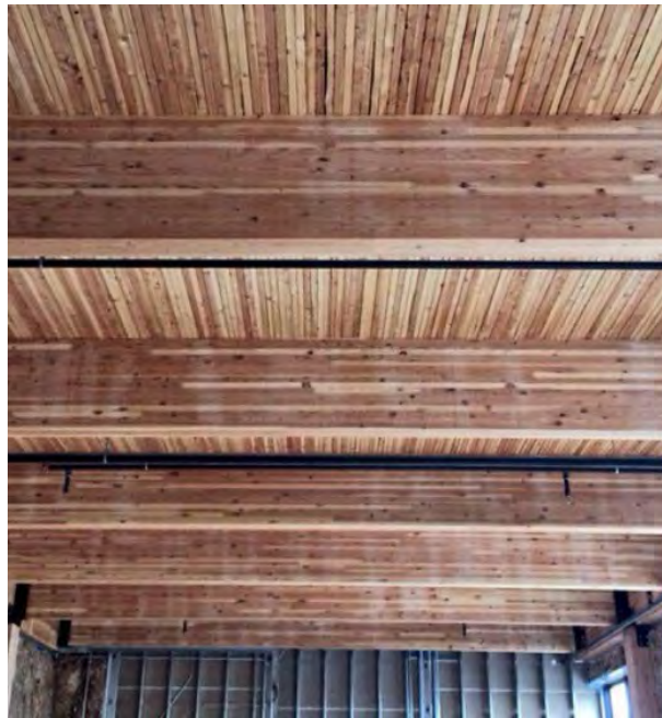
Figure 5.1: NLT and Glulam Girder System
