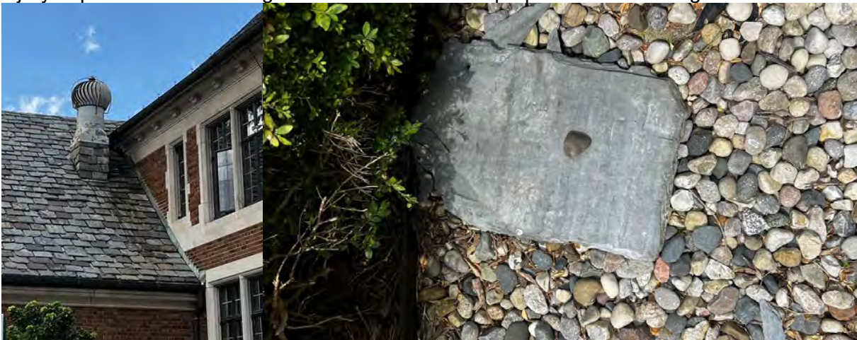
IMAGES 3.1.19 SLATE ROOF
