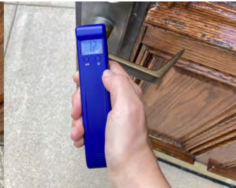
IMAGE 4.2.04 EAST SIDE ENTRY DOOR
