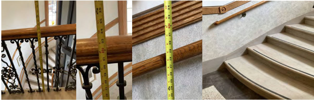
IMAGE 4.2.11 - CENTER STAIR RAILING
