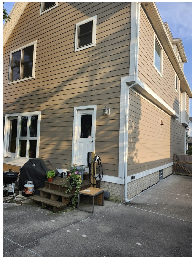
Context of rear door and landing relative to scale of house.
