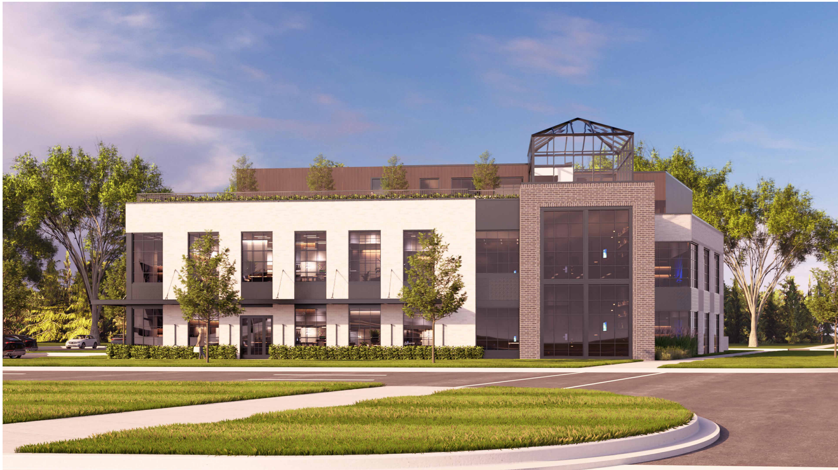
View of East facade from Woodward Avenue
