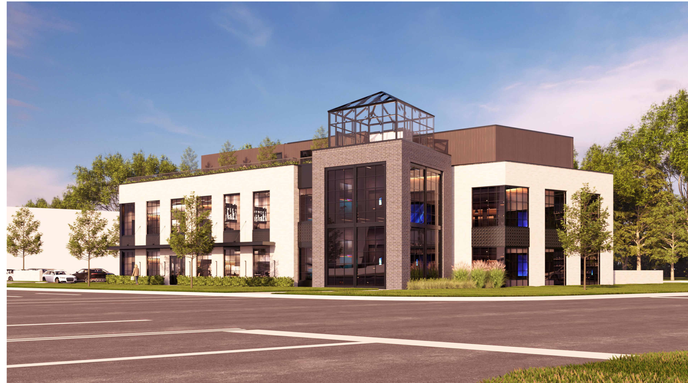
View of Northeast facade from intersection of Woodward Avenue and Quarton Road
