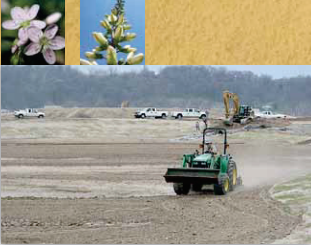
Site preparation for wetland mitigation, Cincinnati, OH
