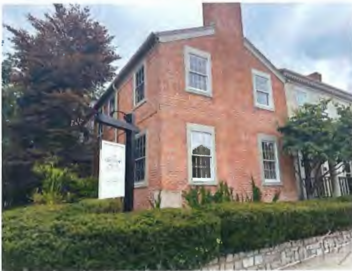
The Community House 380 S. Bates St. Birmingham, Michigan
