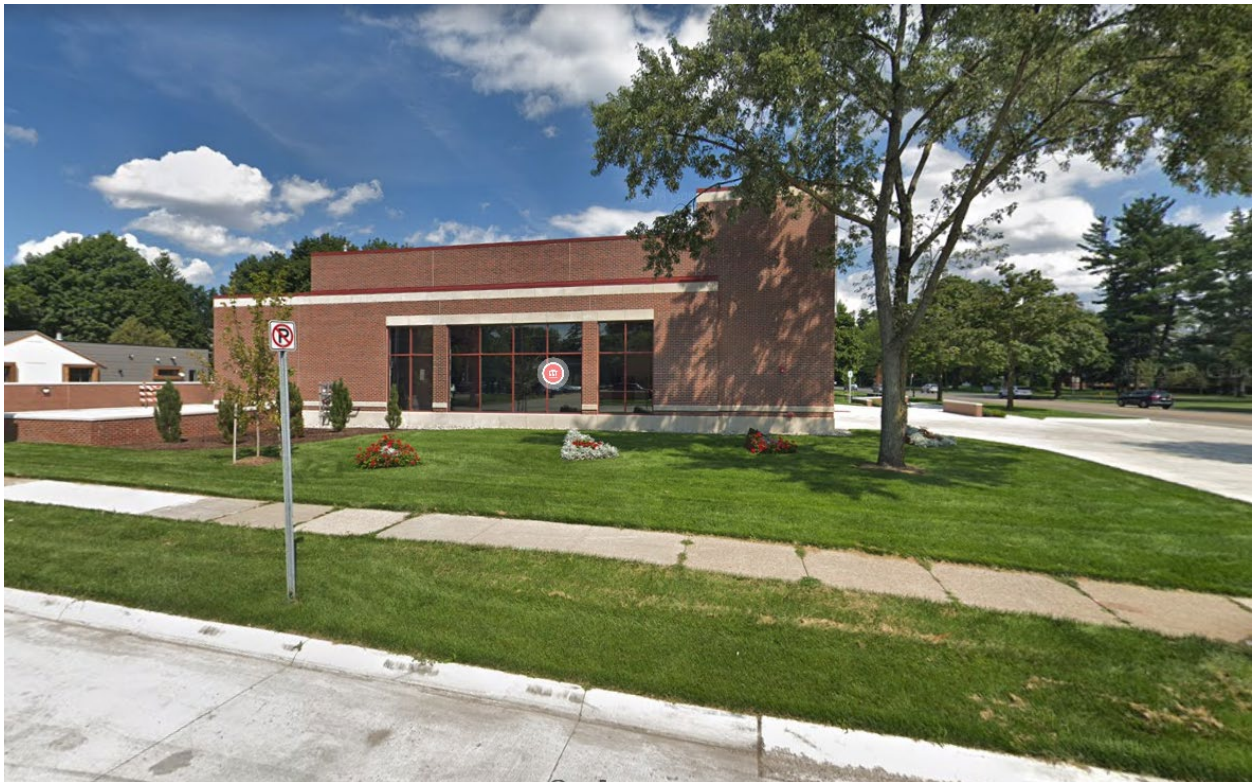
West Side of Chesterfield Fire Station
