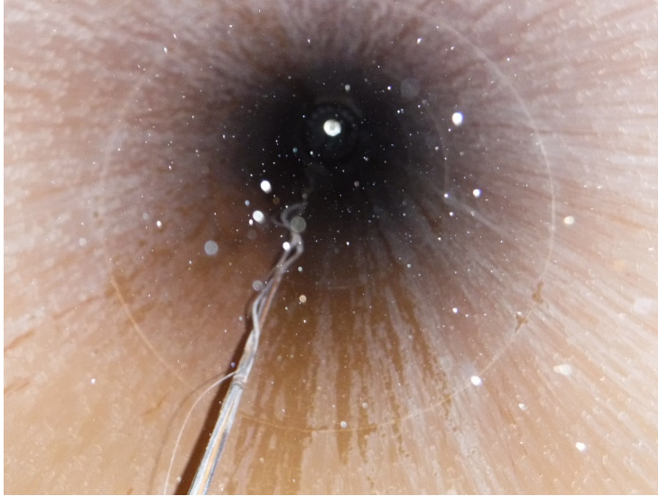
58) The cathodic protection system through the riser is in good condition.
