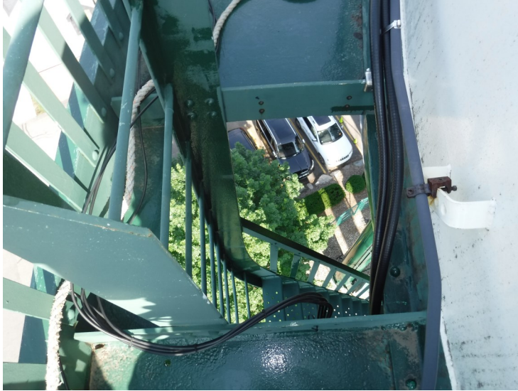
19) There is no cover over the ladder opening in the balcony.
