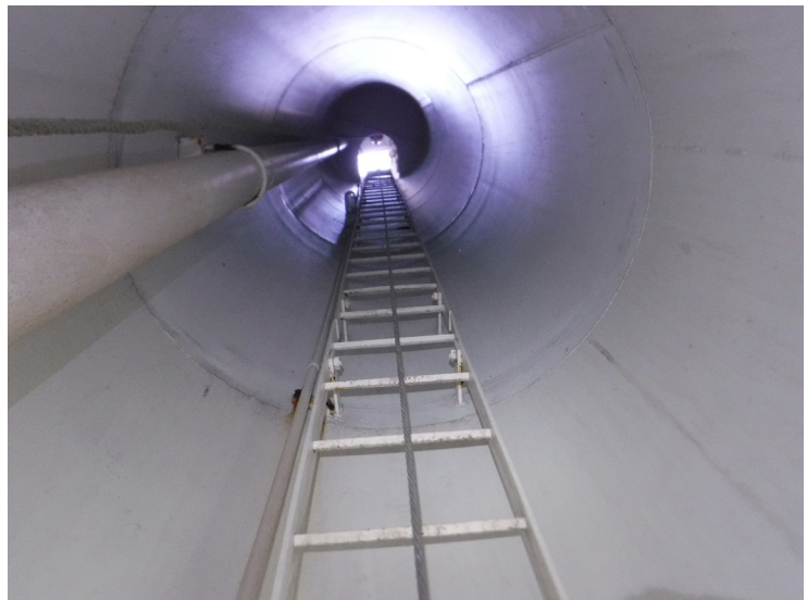
38) The access tube is coating is in good condition overall. The access tube ladder is in good condition. The ladder is equipped with a fall prevention device.
