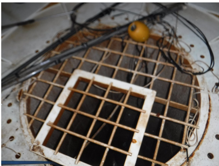
54) The riser is covered with a grate that has an opening. The opening is not hinged.
