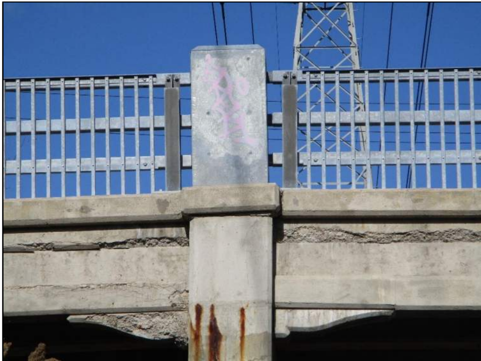
Deterioration on south fascia with out of plumb steel railing post at west pier
