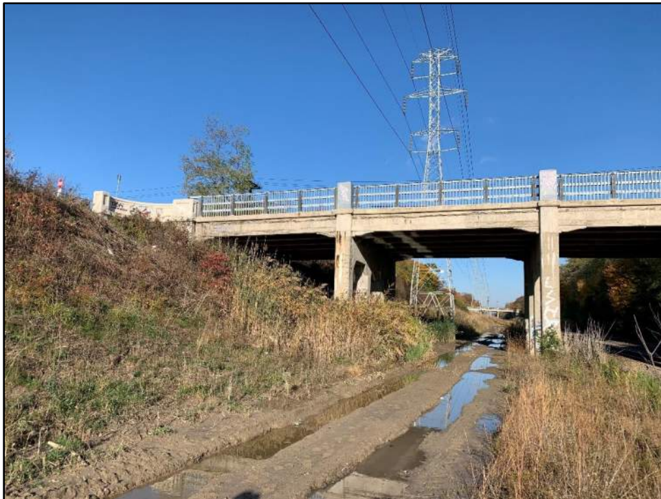
South elevation - west portion
