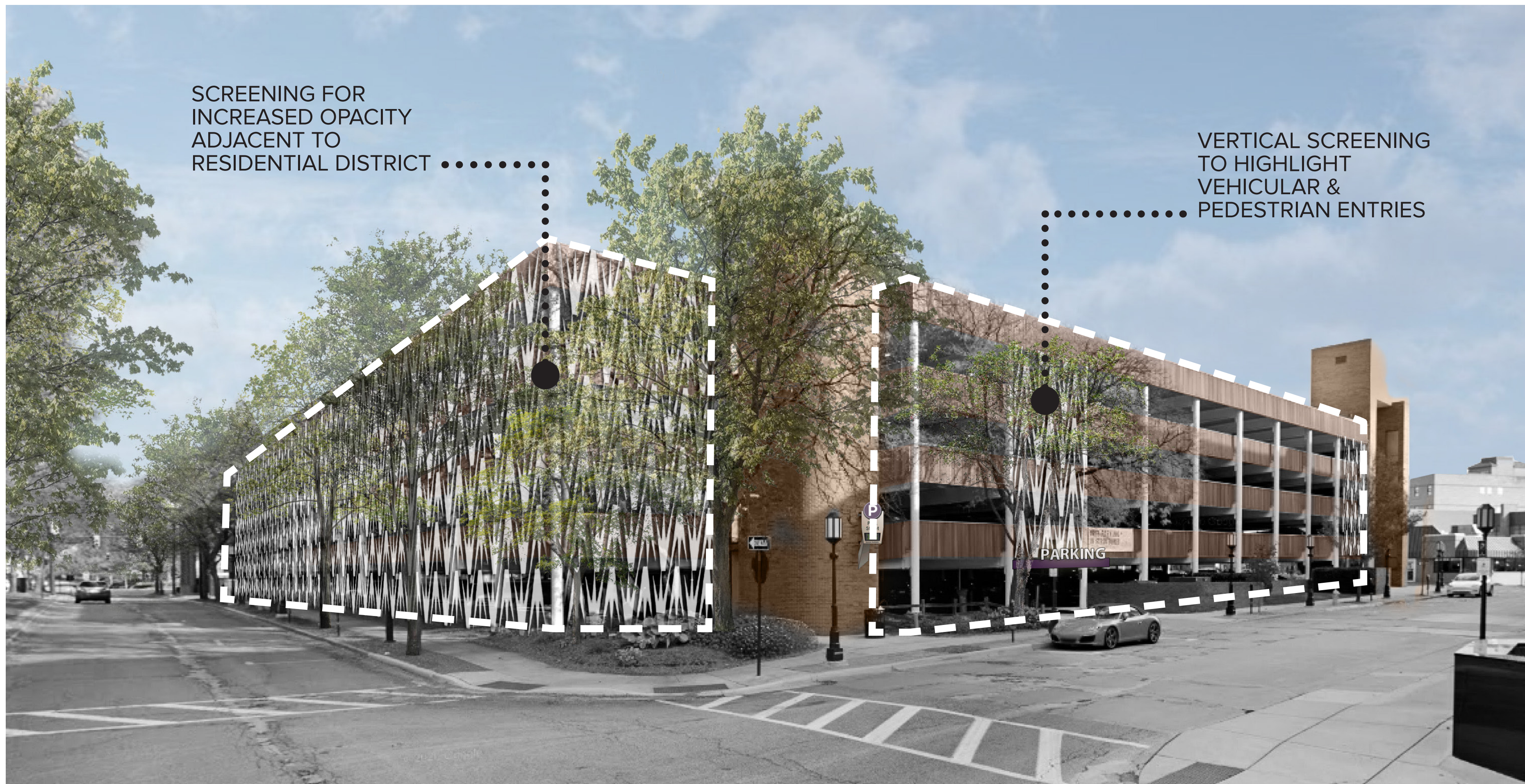
FACADE 2 - REPLACED ALUMINUM PANELS W/ PATTERNED SCREENING
