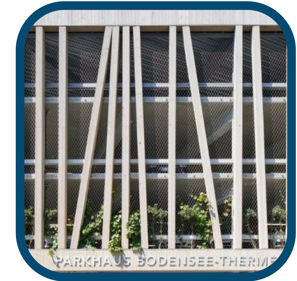
ANGLED FACADE SYSTEM PROVIDES IRREGULARITY & INTEREST
