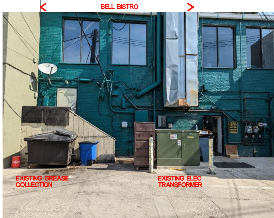
Image B - Rear Alley | Transformer/Utilities
