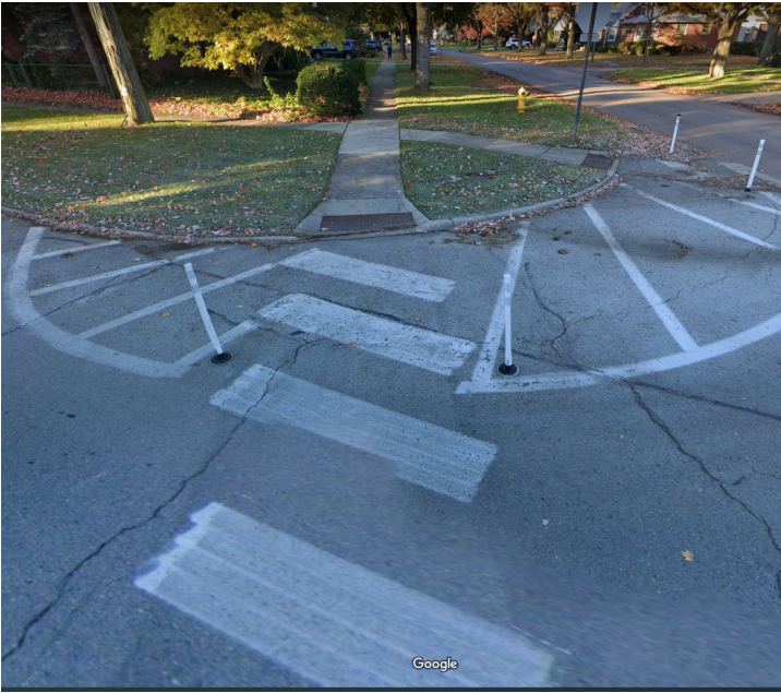
Existing painted bumpouts and bollards
