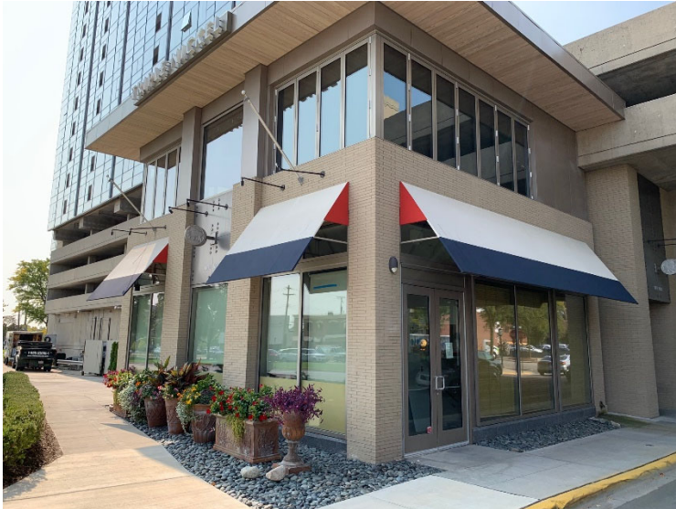
Existing Awnings – SW Corner
