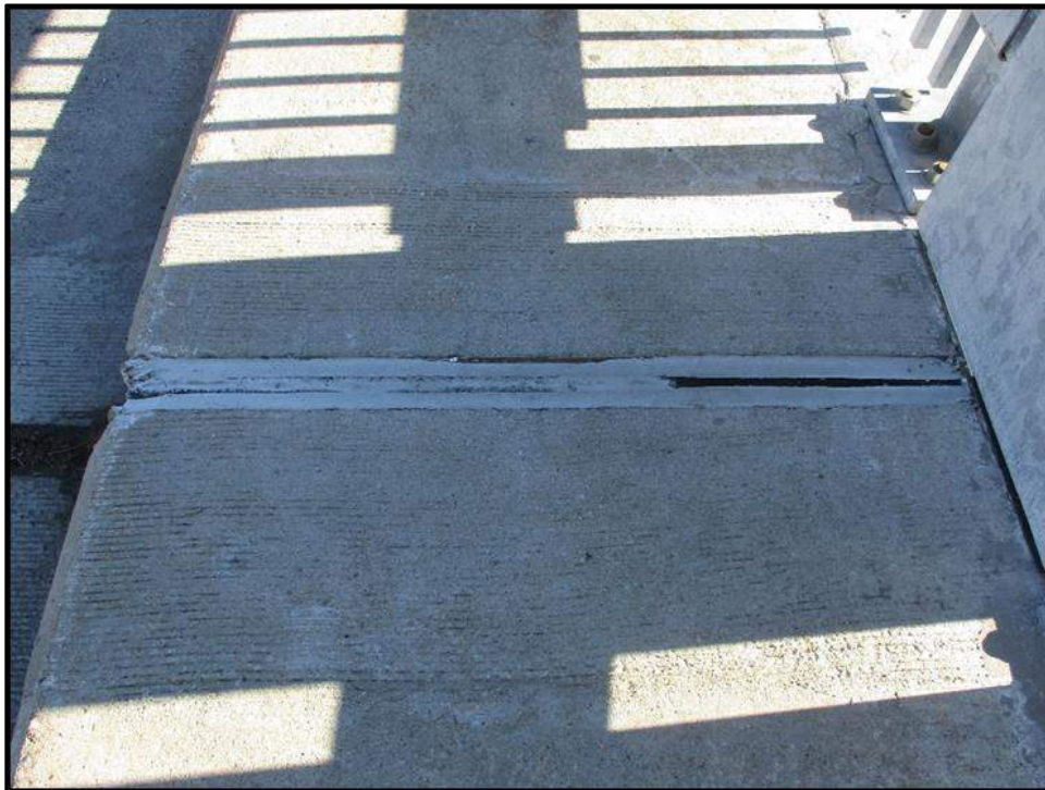
Separation of sealant at south sidewalk expansion joint
