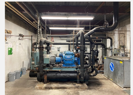
Mechanical Rm. Before
