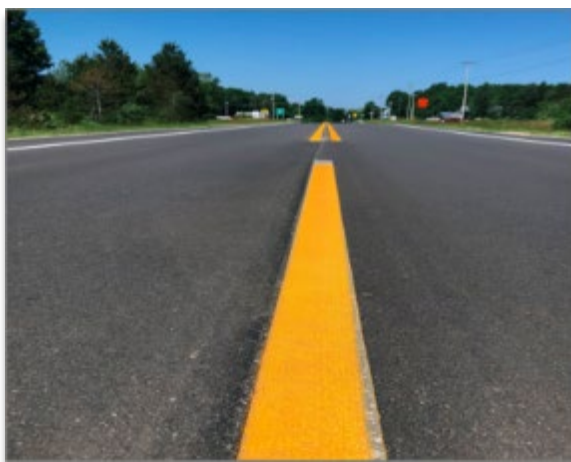
Retroreflective Pavement Markings 8
