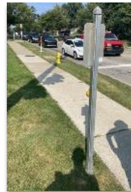
Improper Placement of a Push Button
