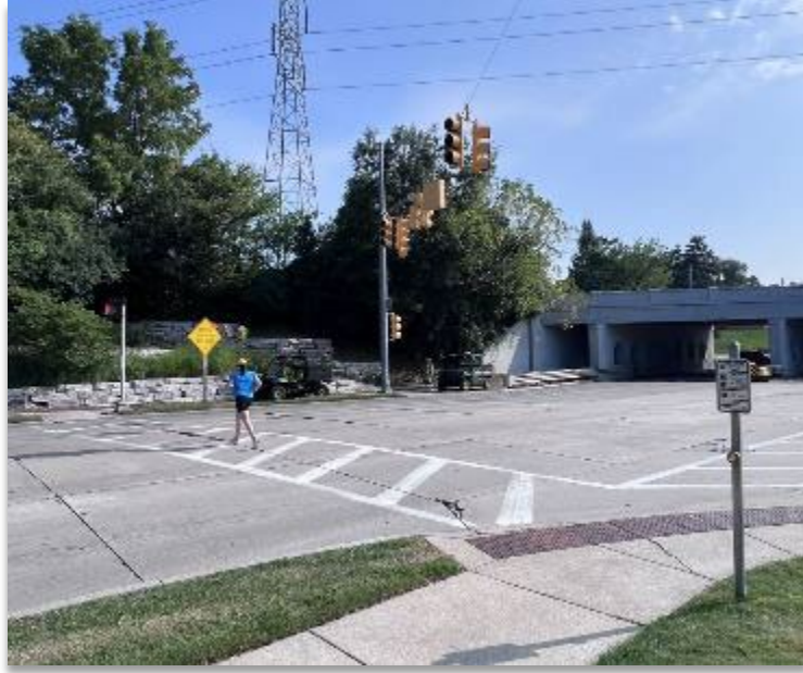
Figure 24 - Diagonal Span Configuration at Maple Road and S. Eton Street
