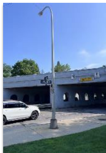
Light Pole Within the Sidewalk
