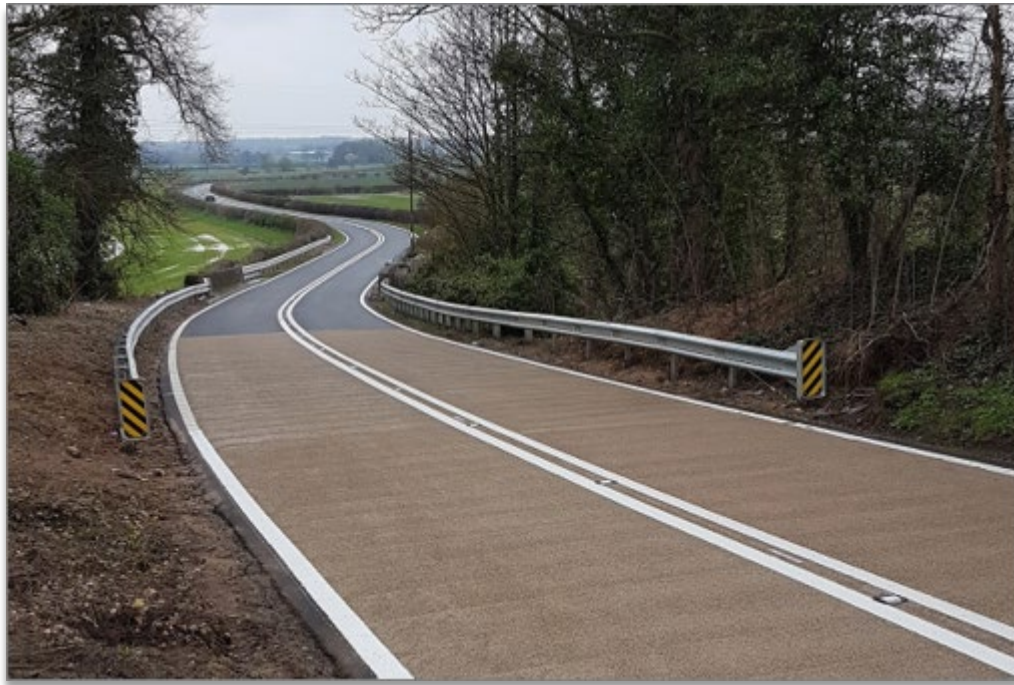
Figure 22 – Example of the High Friction Surface Treatment (HFST) 7
