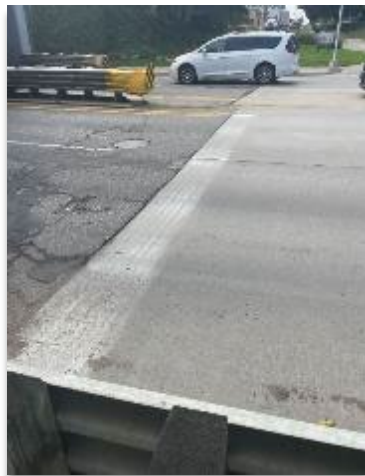
S Eton Street Westbound Stop Bar
