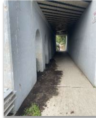
Sidewalk under the Viaduct
