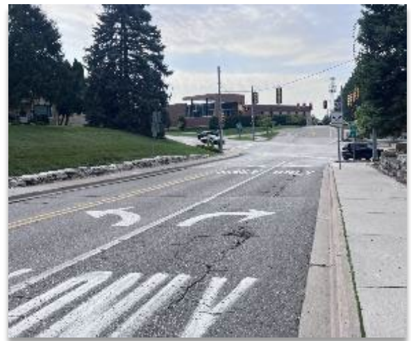
Lane Marking and Supplemental Lane Signage
