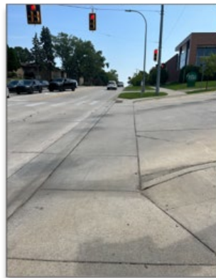
Whole Foods Driveway Crosswalk
