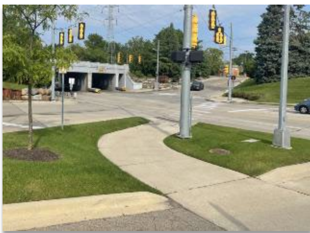
Jog in the Sidewalk at Whole Foods Driveway
