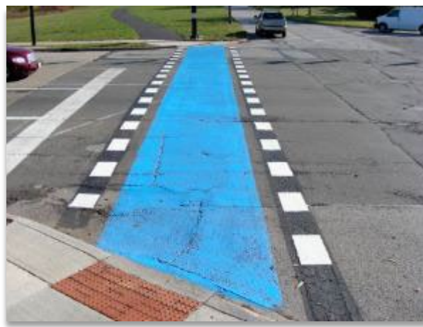
Methyl Methacrylate (MMA) Pavement Markings 9
