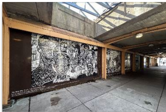
Figure 34 – Decorative Viaduct with Mural Panels and Lighting in Chicago, Illinois 12
